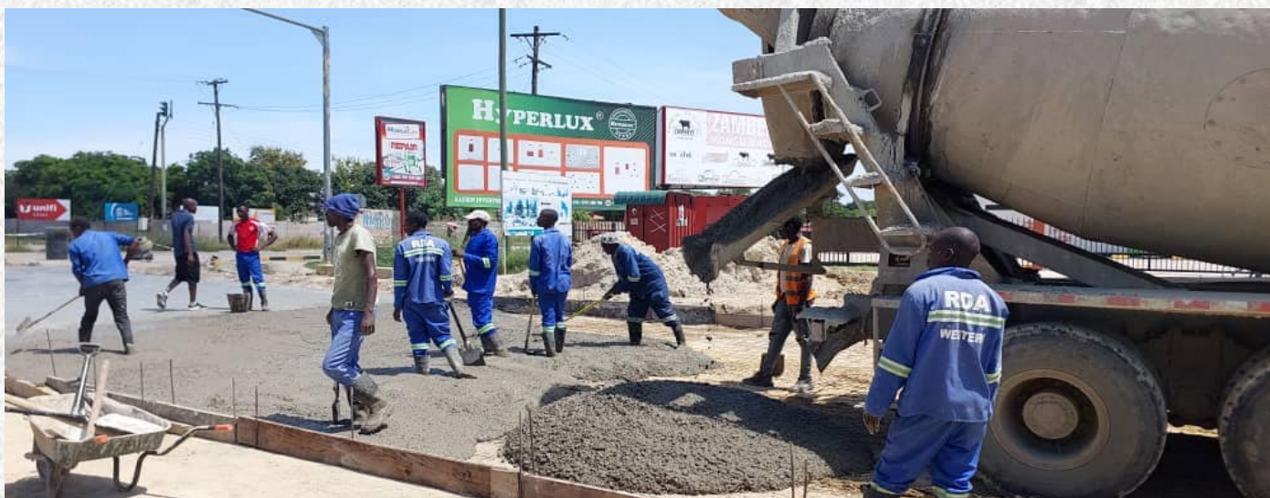
The construction of a 60 meters rigid pavement at Mongu traffic lights.
