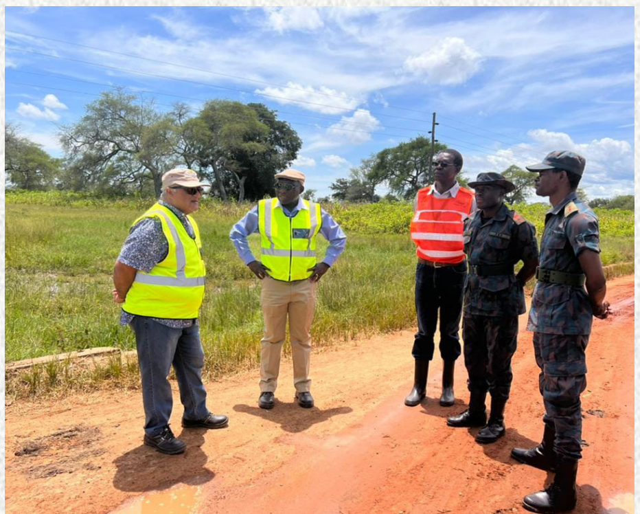
Minister of Infrastructure Housing and Urban Development, Hon. Eng. Charles L. Milupi (second from left) and Road Development Agency (RDA) Board of Director Chairperson, Eng. Mulchand Kuntawala being briefed on the progress achieved on works on the Monze-Niko road by the Zambia National Service (ZNS) Southern Province Commander, Col. Richard Chanda (second from right) during the inspection of the road.
