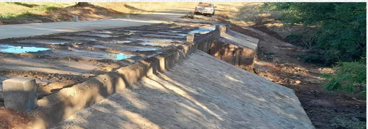
Mthiko Culvert after the works.
