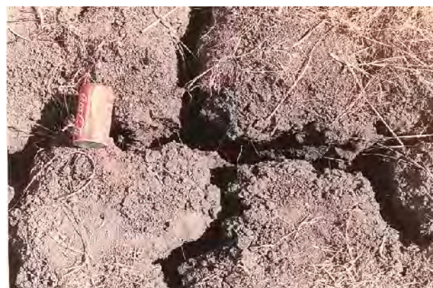
Figure 4-7: Cracking on expansive clays
