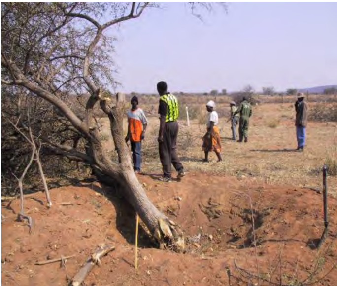
Figure 13-5: Tree removal and de-stumping
