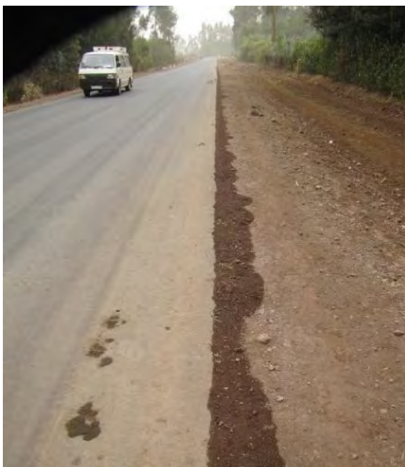
Figure 8-4: Infiltration of water through a permeable surfacing
