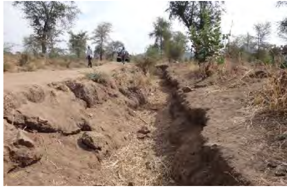
Figure 4-14: Gully formation in erodible soil
