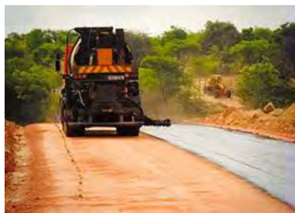
Figure 1-1: Construction of a LVR in Zambia
