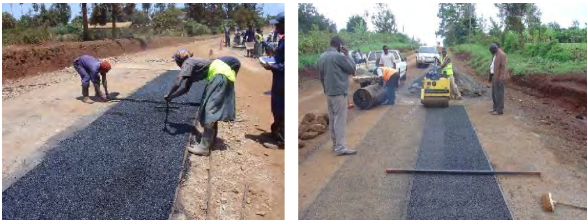
Figure 11-7: Levelling and compaction of CMA
