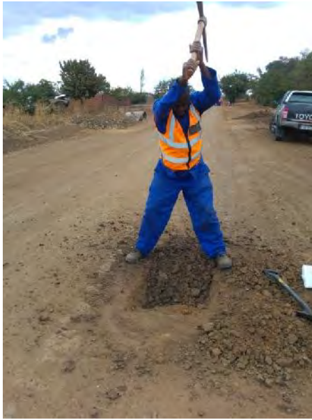
Figure 4-4: Excavation of test pit by hand
