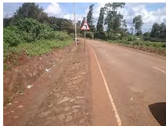
Figure 8-19: Good – Drain lining connected to edge of surfacing
