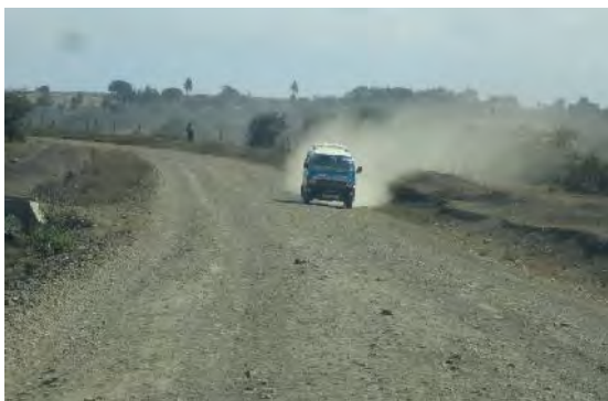
Dusty and rough due to oversize material
