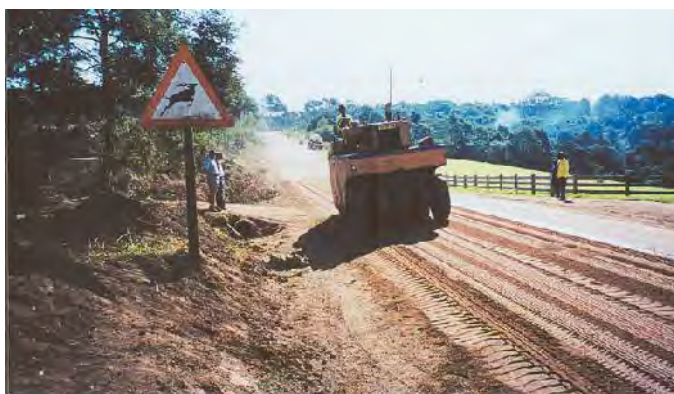
Figure 11-6: Extensive rolling of an Otta Seal is essential to achieve a good result
