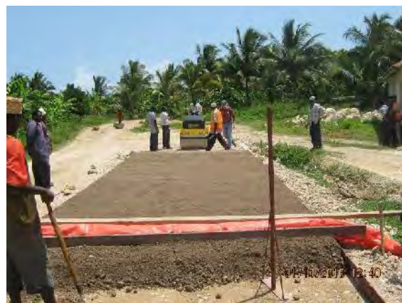
Figure 13-4: Shutter system for construction of ETB base by LBM
