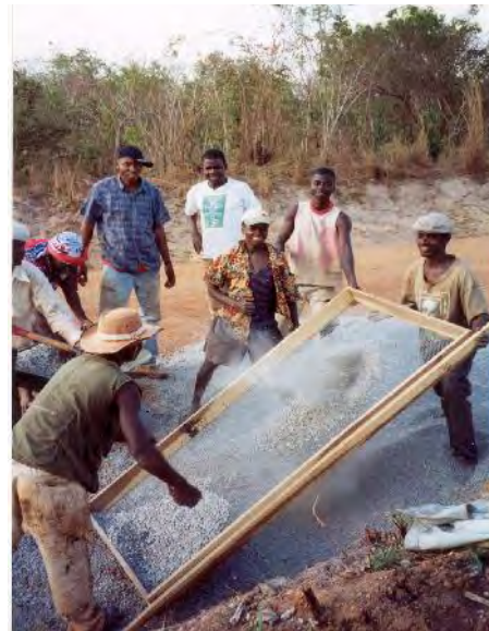
Figure 13-6: Screening of aggregates
