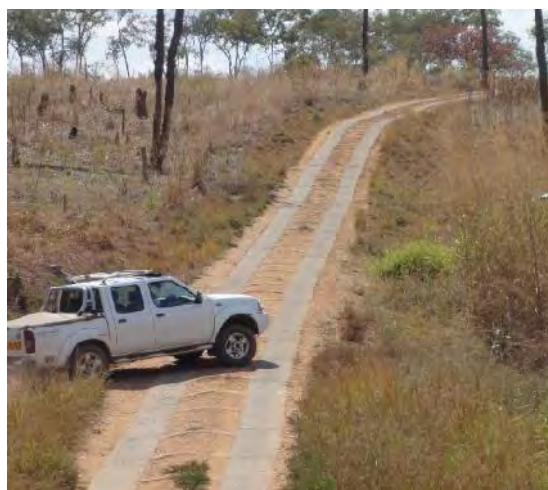
Figure 9-16: Concrete strips to provide access up a steep, sandy section
