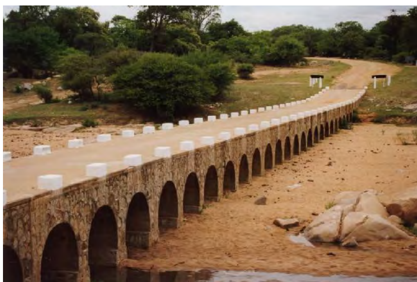
Figure 7-10: A typical vented drift/causeway
