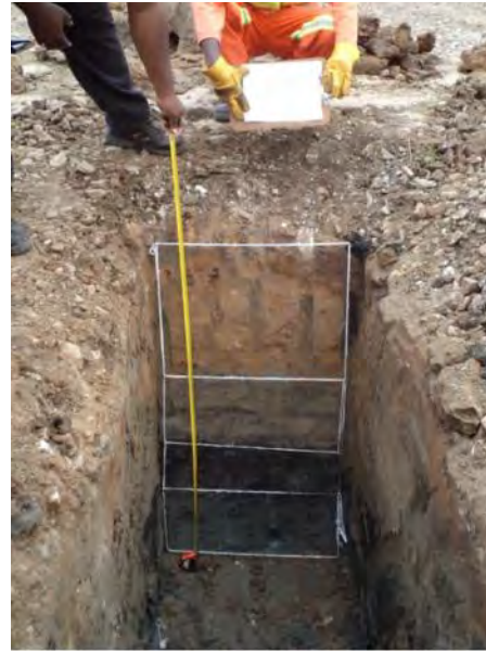
Figure 4-5: Logging of subgrade layers
