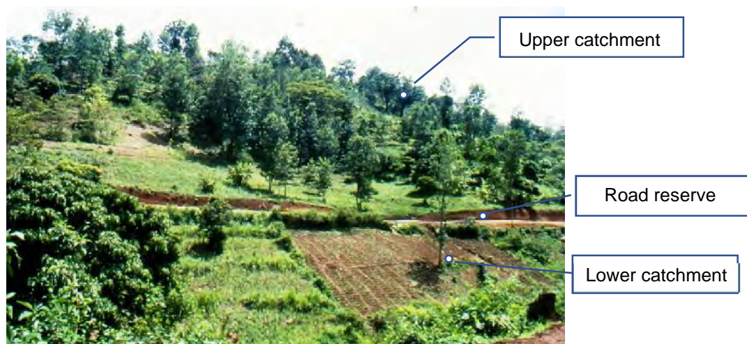
Figure 8-14: Erosion areas—upper catchment, road reserve and lower catchment
