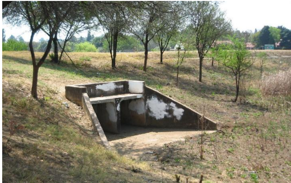
Figure 5-1: Attenuation dam and inlet to outlet structure
