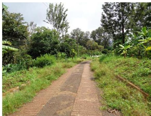
Figure 2-8: Example of poorly maintained concrete strip road
