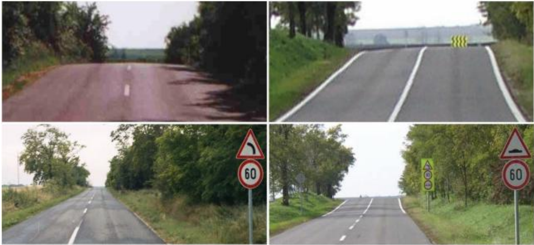
Figure 2-6: Use of edge markings to improve road safety on vertical crest curve
