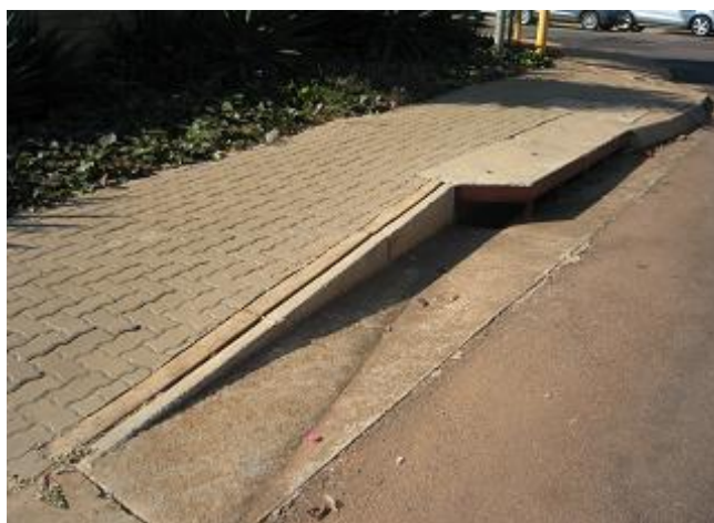
Figure 5-4: Kerb inlet
