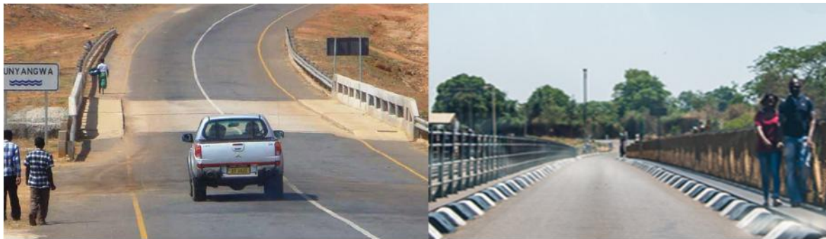
Figure 4-22: Long bridge with separate walkway
