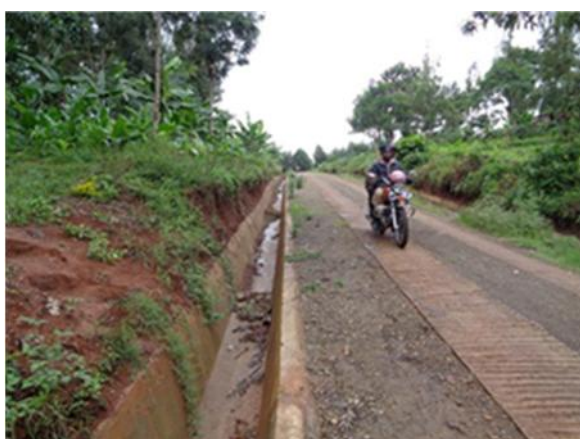
Inappropriate design of side drain
