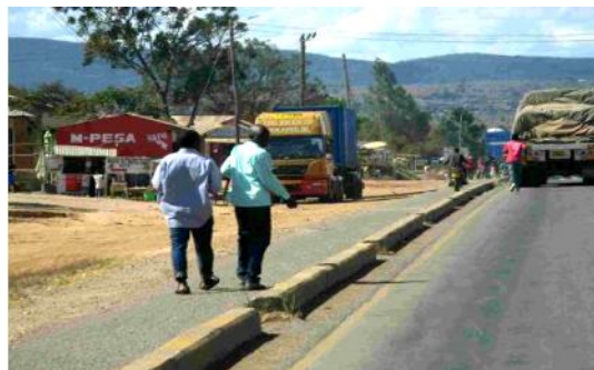
Segregated shoulder using barrier kerb
