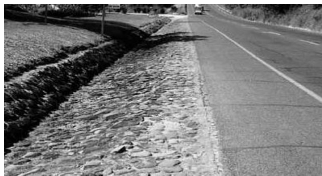
Figure 5-5: Undesirable drain design
