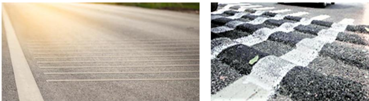
Figure 4-3: Examples of well designed (left) and poorly designed (right) rumble strips
