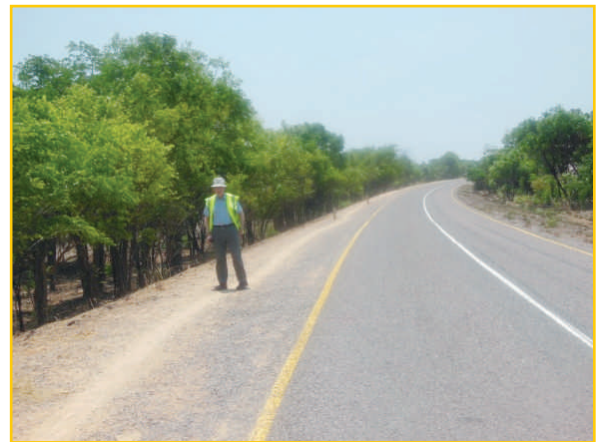
Completed section of Mansa Nchelenge
