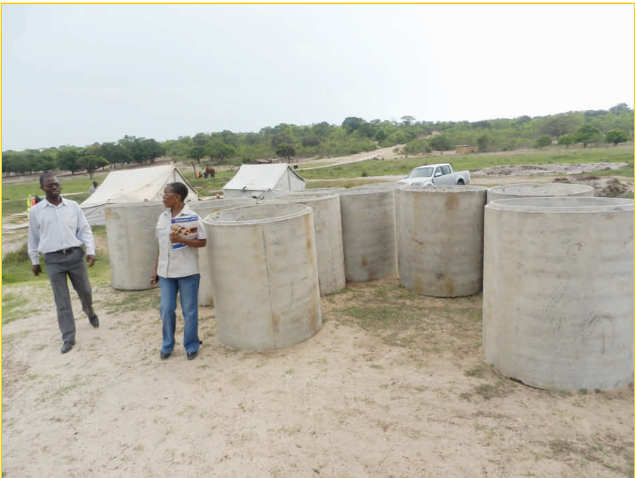
Audit inspection of culverts
