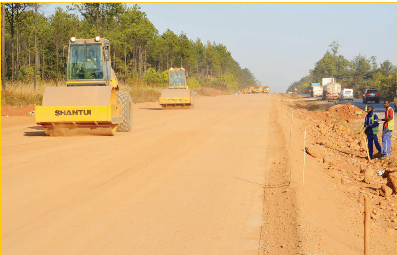
Construction works on Kitwe-Chingola dual carriageway
