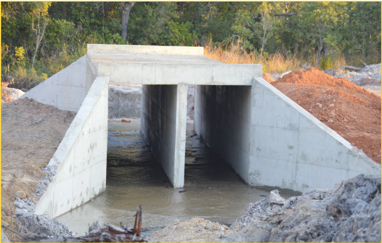
Box Culvert under construction
