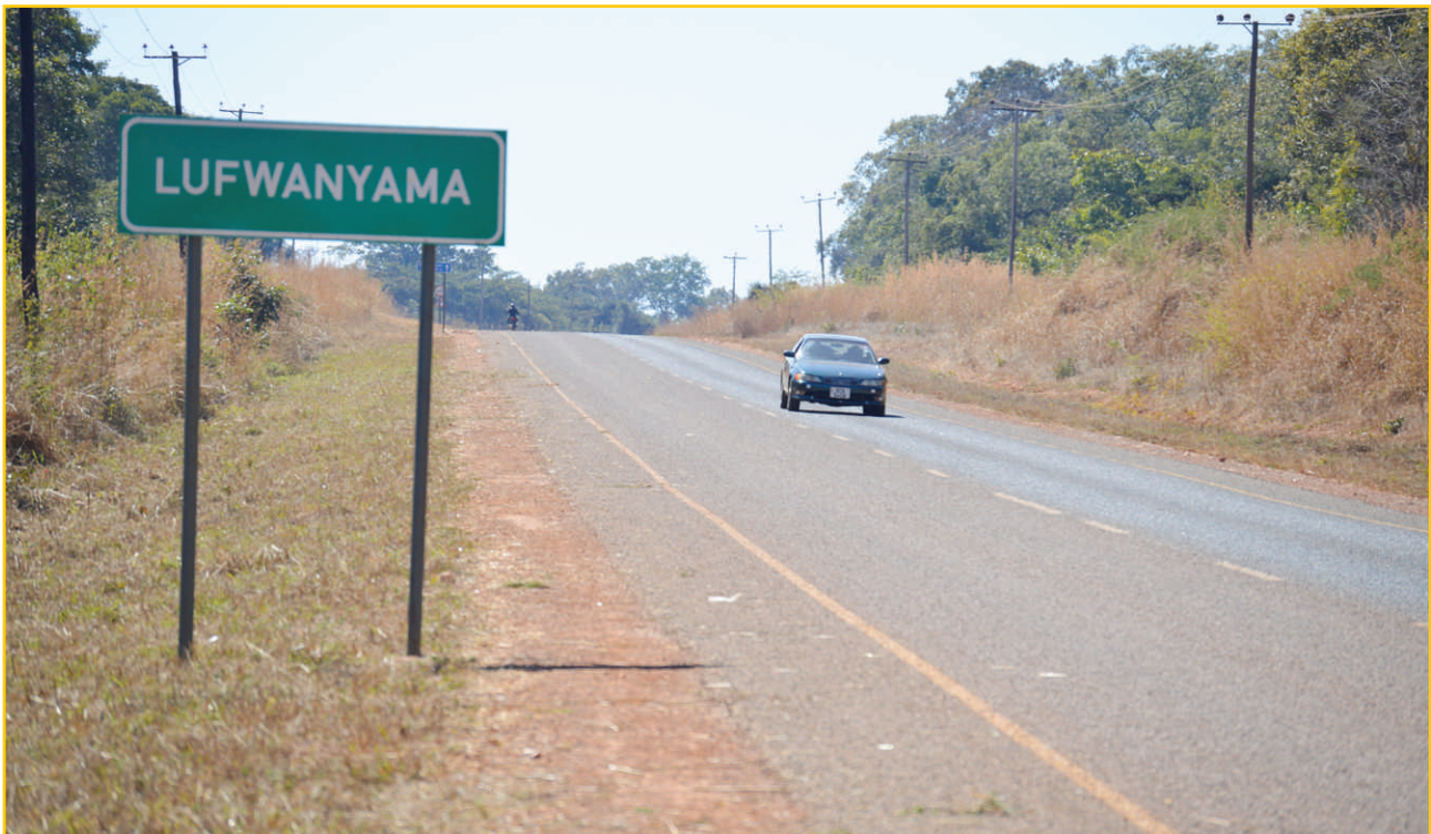
Completed section of the Kalulushi-Lufwanyama Road
