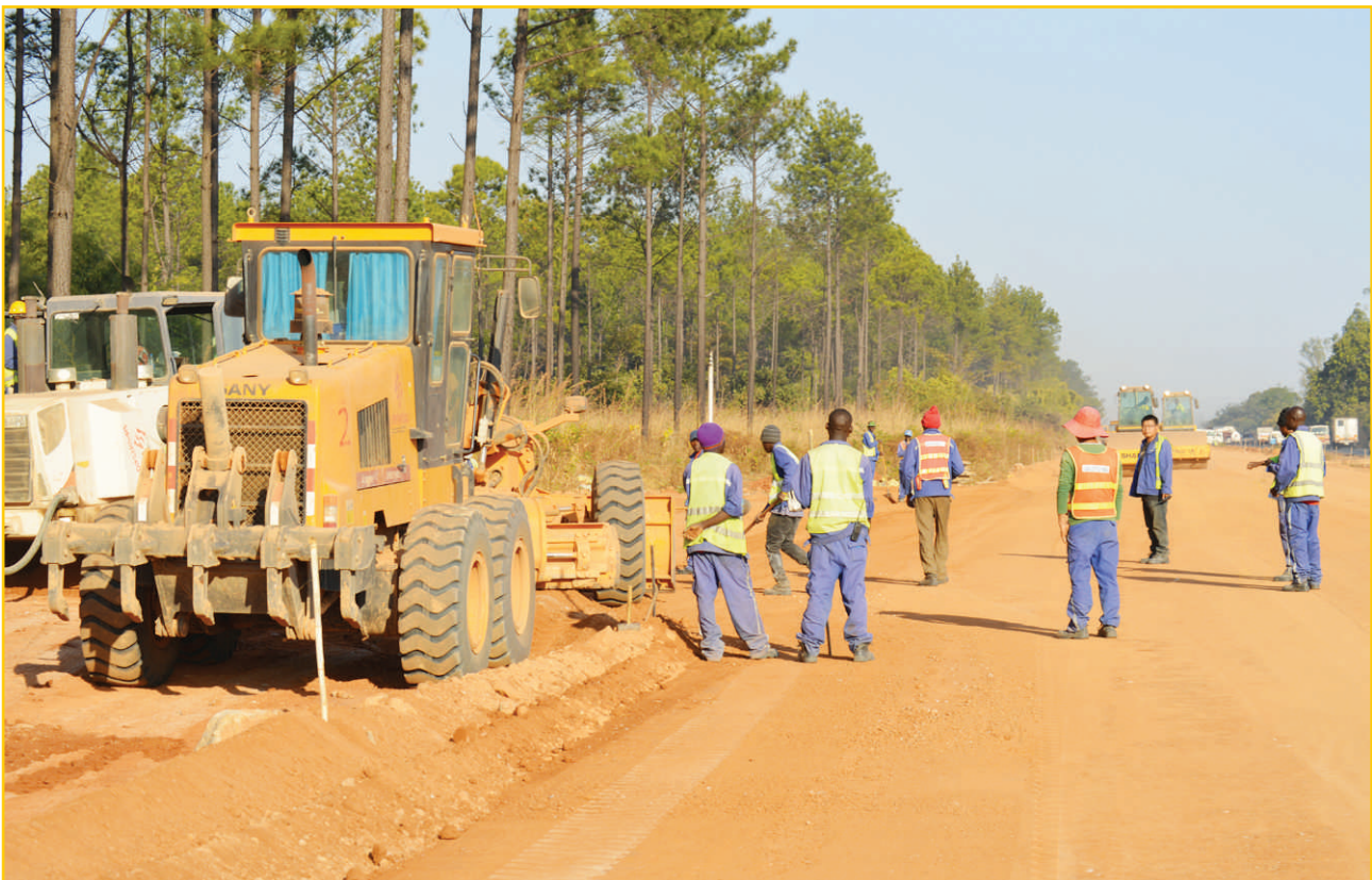
Construction works on Kitwe-Chingola dual carriageway
