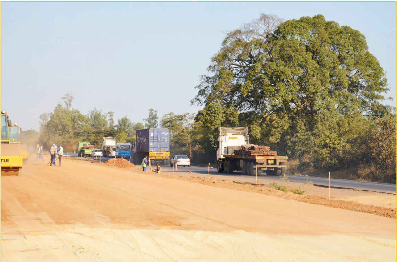
Works on Chingola – Kitwe dual carriageway
