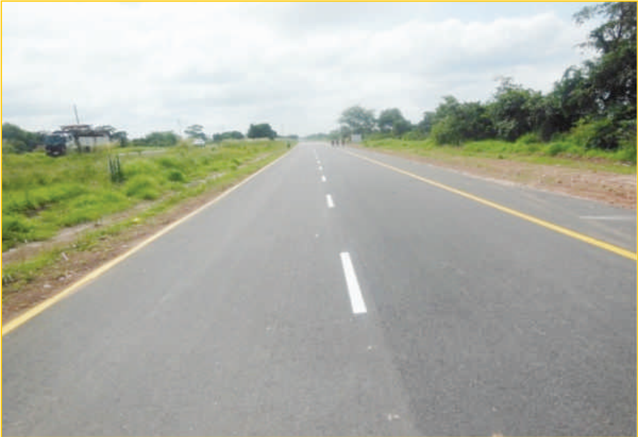
Completed section of the Ndola-Kitwe Dual Carriageway
