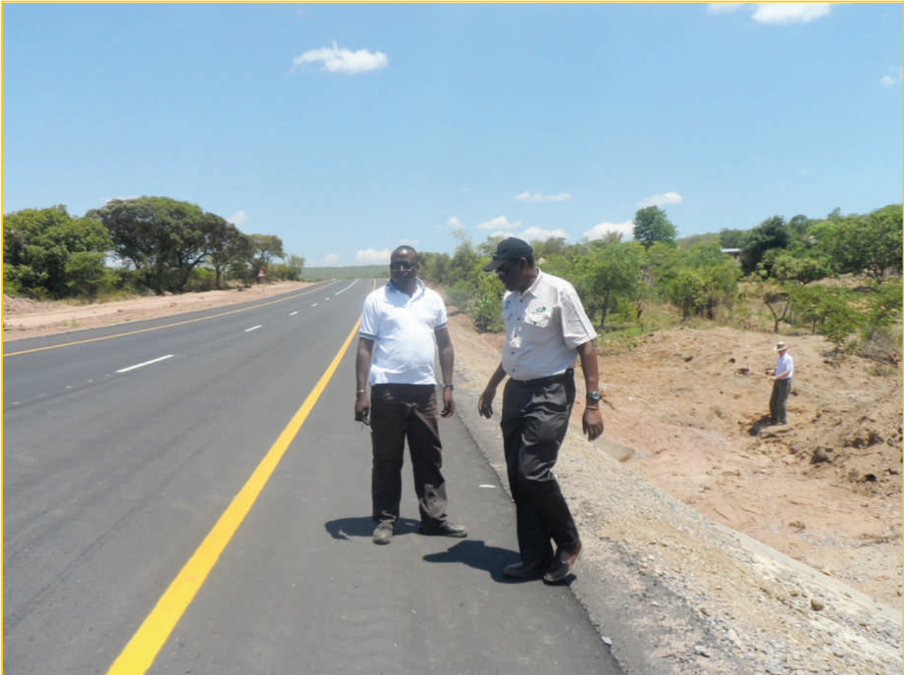
Inspection of Lusaka – Chirundu Road works
