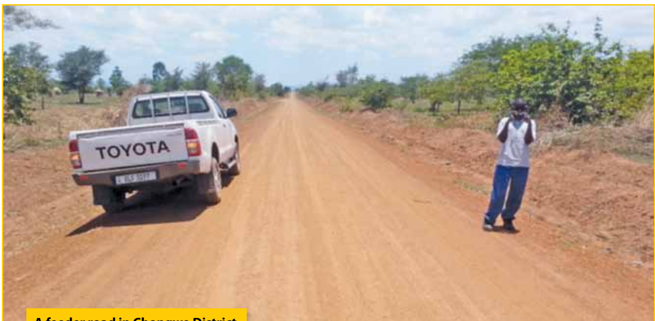
A feeder road in Chongwe District
