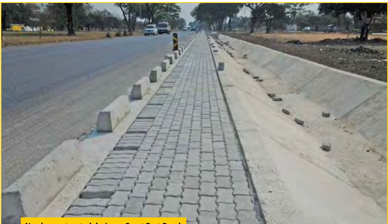
Newly constructed drain on Great East Road
