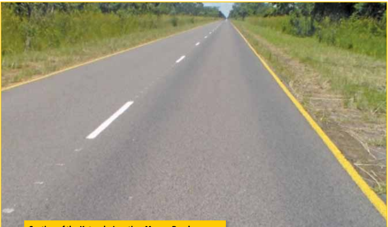
Section of the Katunda Junction-Mongu Road
