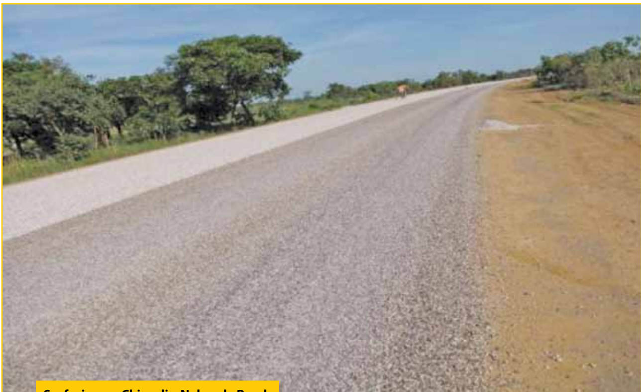
Surfacing on Chinsali – Nakonde Road
