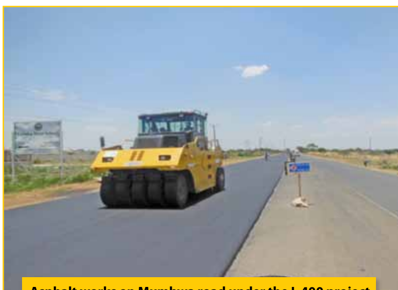
Asphalt works on Mumbwa road under the L 400 project
