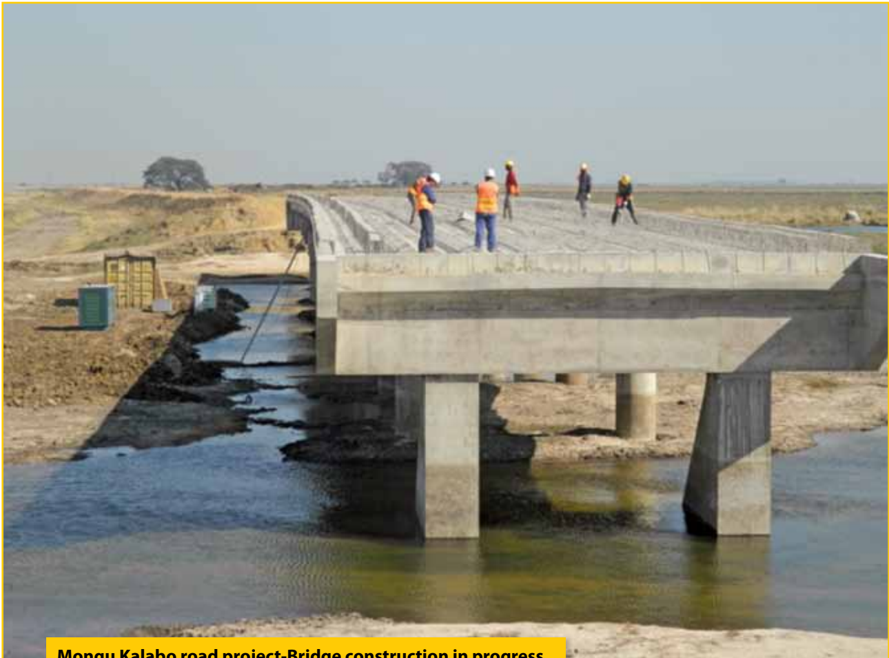
Mongu Kalabo road project-Bridge construction in progress
