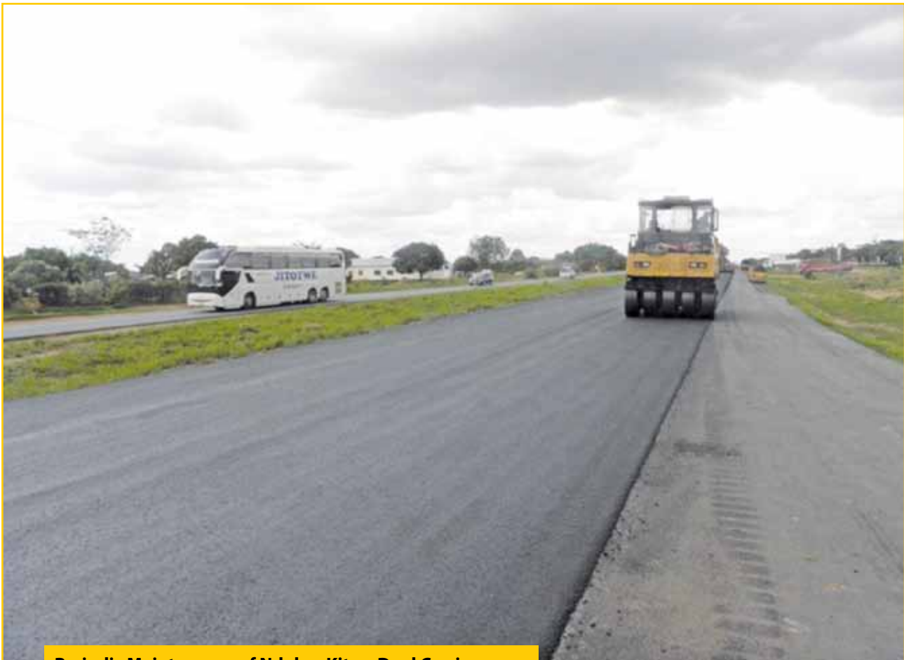
Periodic Maintenance of Ndola – Kitwe Dual Carriageway
