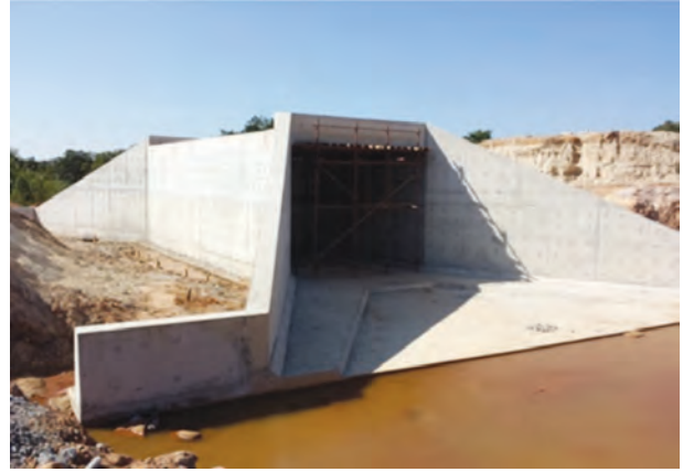
Figure 10: Box culvert under construction
