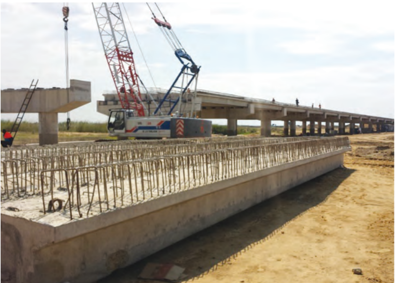
Figure 11: Bridge works in progress-Mongu-Kalabo Road
