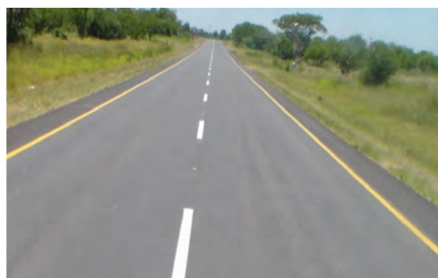
Figure 13: Completed Section of Livingstone to Sesheke road (M10)
