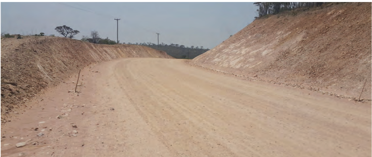
Figure 4: A typical cutting through a mountainous section during road construction
