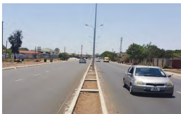
Figure 12: Newly constructed Chilimbulu Road
