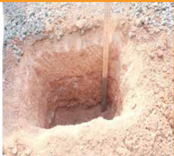
Figure 3: Chipata Mfuwe - Measuring thickness of subgrade, Sub-base and road base
