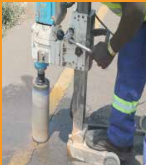
Figure 2: Chipata Mfuwe - Extracting the core to test layer compliance
