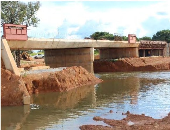
Figure 19: Lubembe Bridge along Pedicle Road
