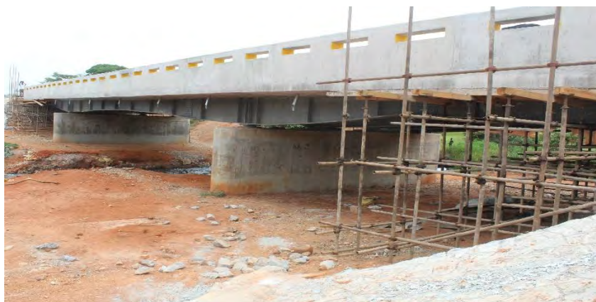
Figure 13: A substantially completed new Mwambashi bridge along the Kitwe-Chingola Road
