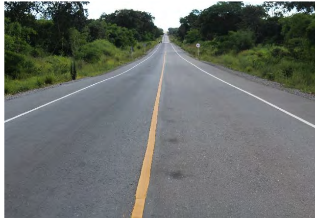
Figure 20: Completed Section of the Pedicle Road
