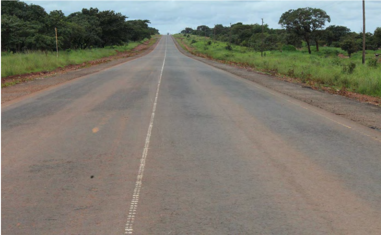
Figure 18: Chingola Solwezi Road under construction
