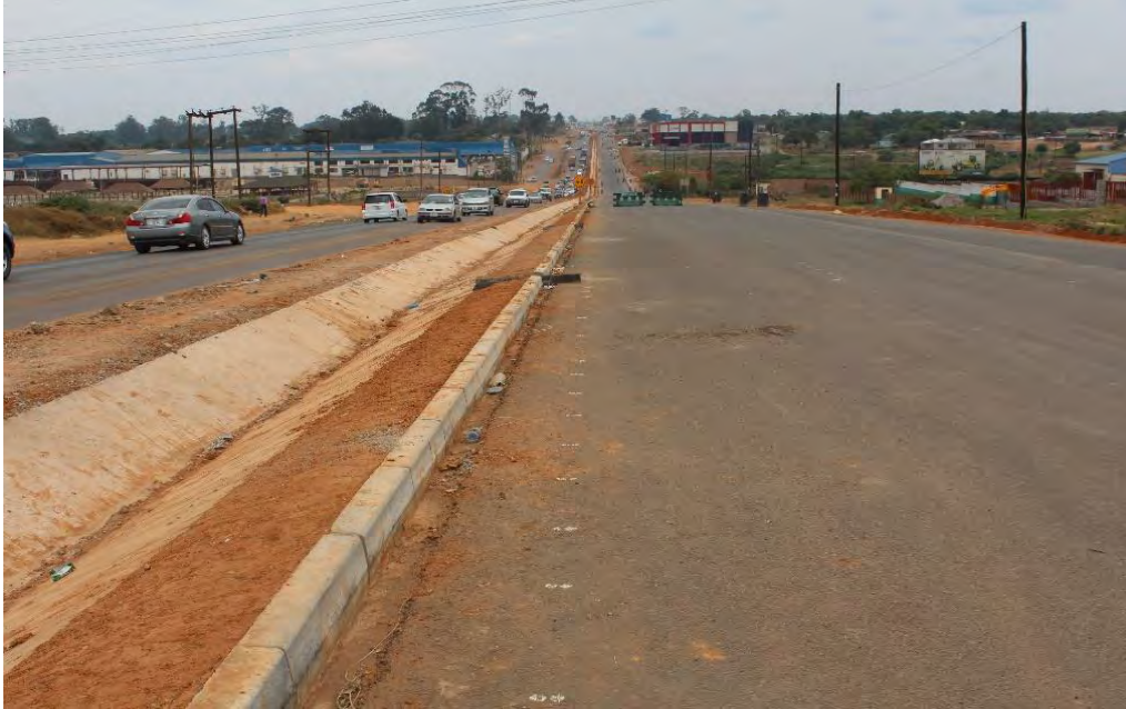
Figure 17: Kitwe-Chingola Dual Carriageway Road under construction
