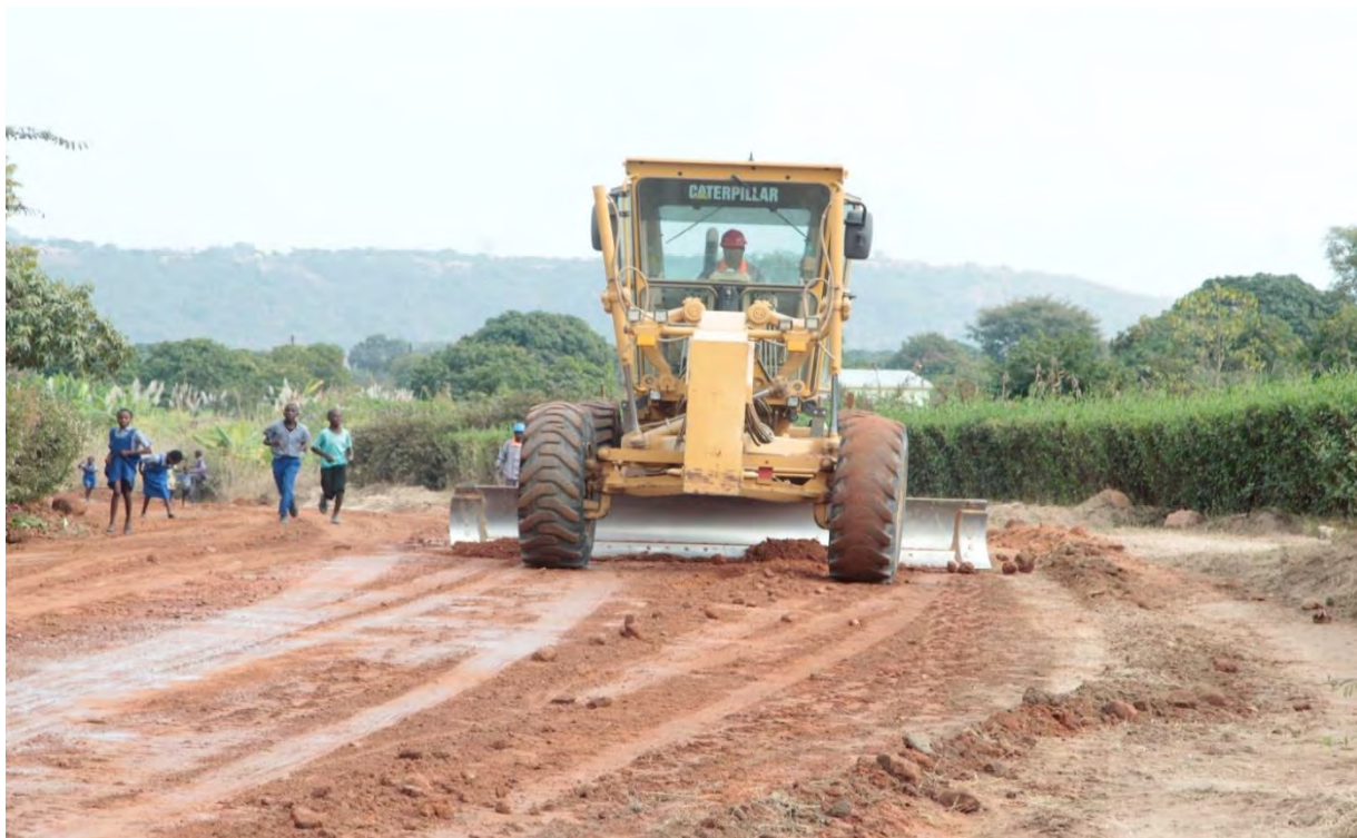
Figure 10: Itezhi Tezhi feeder Road works in progress
