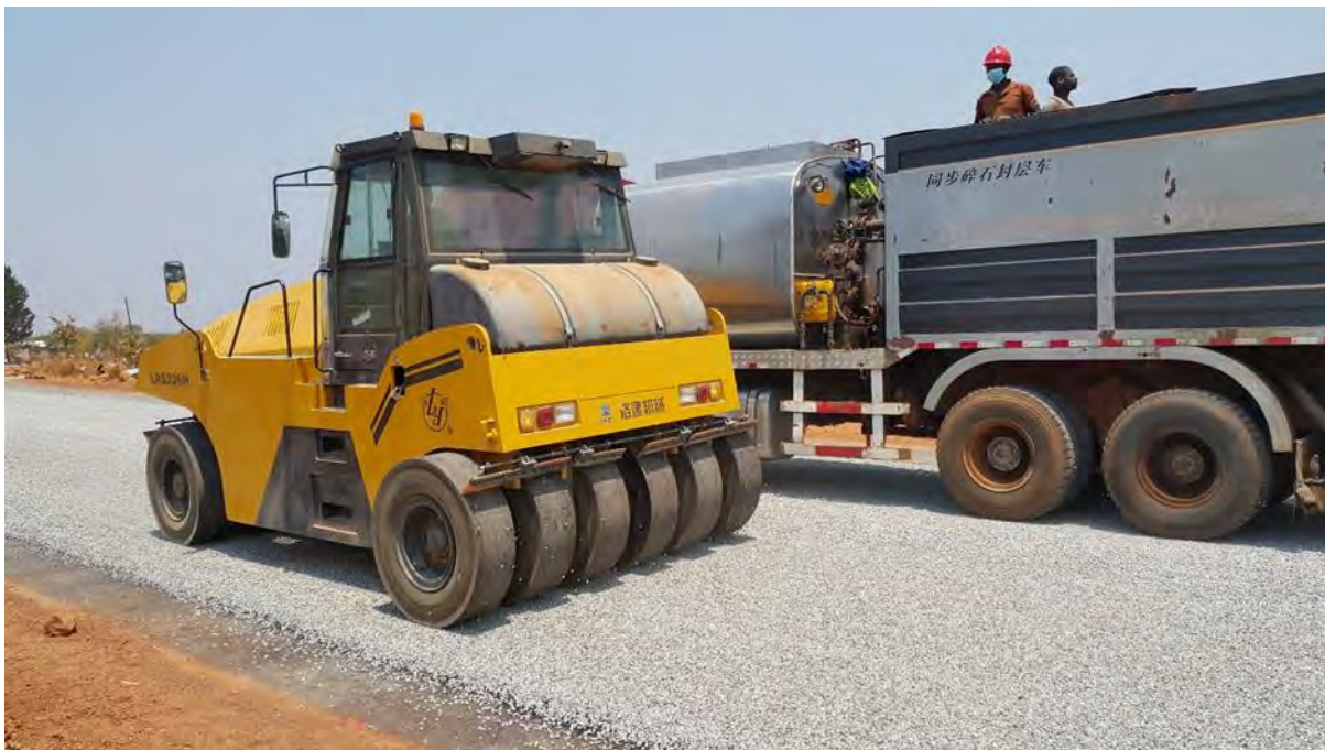
Figure 22: Road Sealing Works in Progress
