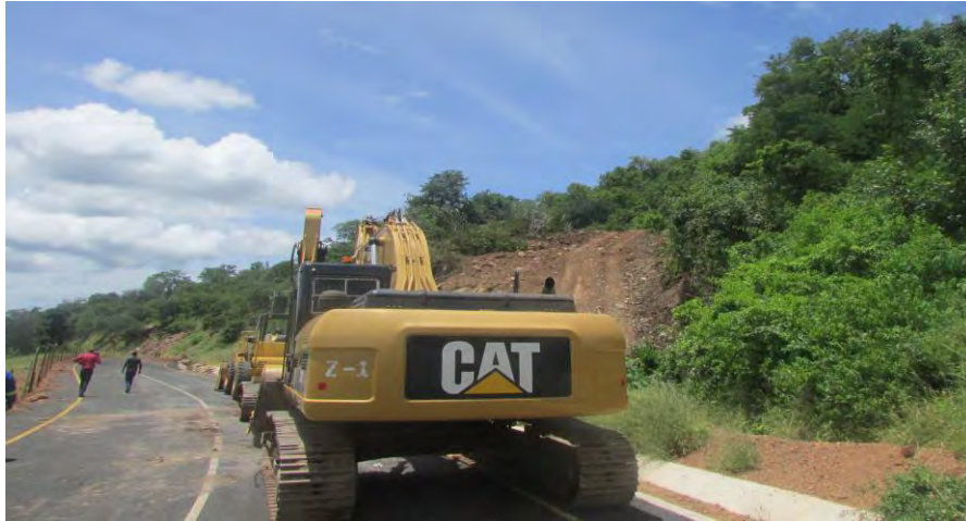
Figure 24: Contractors equipment and Restoration works on site
