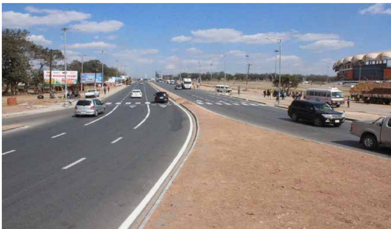
Figure 4: Completed Section of the Great North Road under the L400 Project
