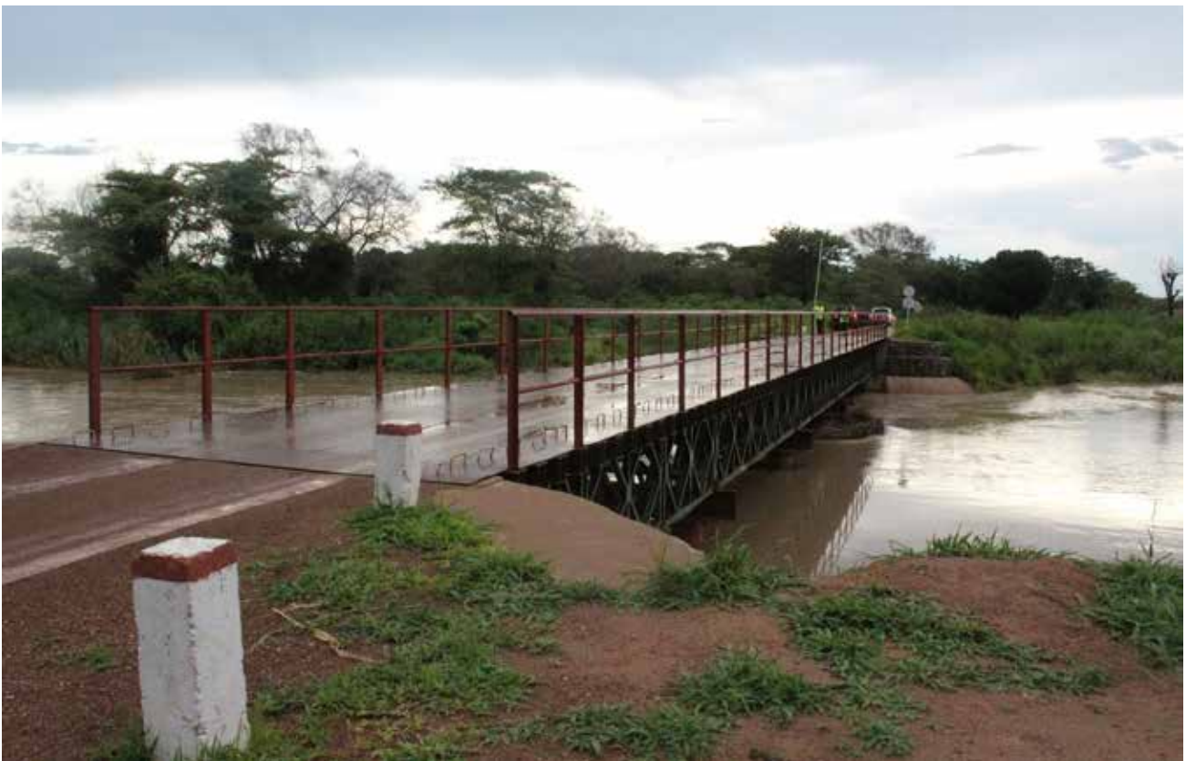
Figure 5: Completed Temporal bridge on Luangwa Matumbo Road
