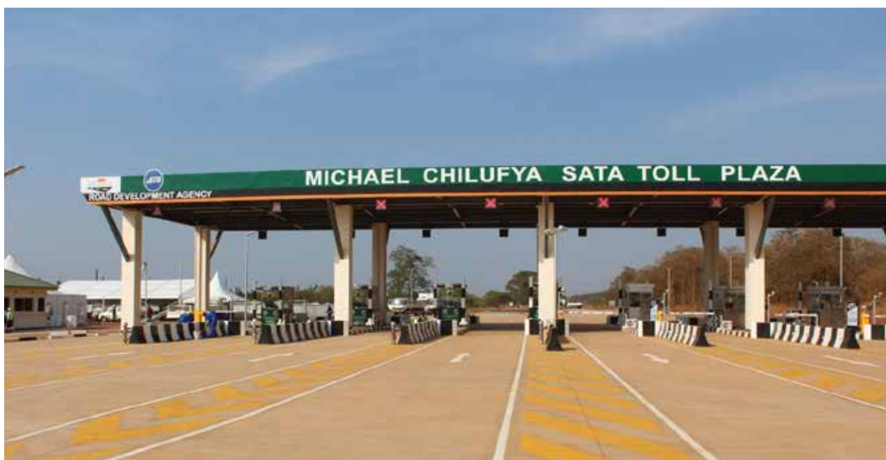
Figure 3: Completed Michael Chilufya Sata Toll Plaza along the Ndola - Kitwe Road
