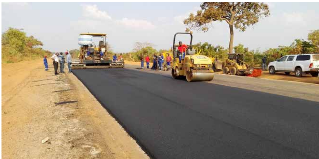
Figure 2: Construction works along Chingola Solwezi road
