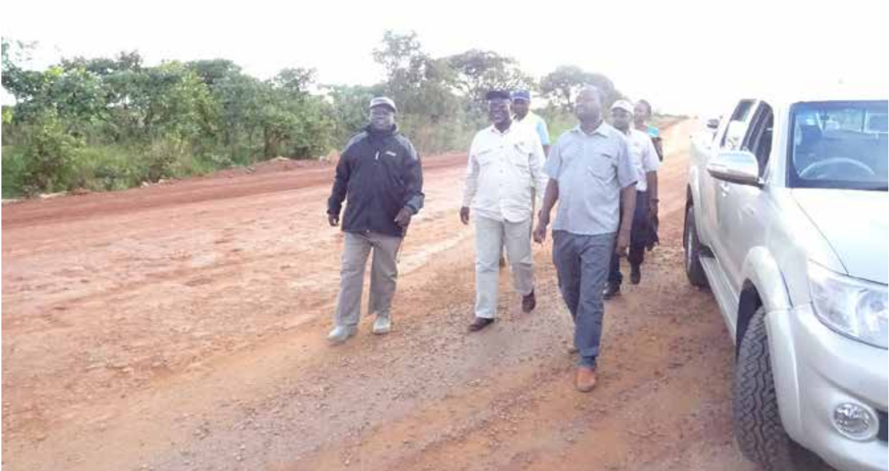
Figure 9: RDA Vice Board Chairperson Eng. Yamfwa Mukanga and Board Member Dr. Mutaba Mwali inspect works at Lukulu Bridge.
