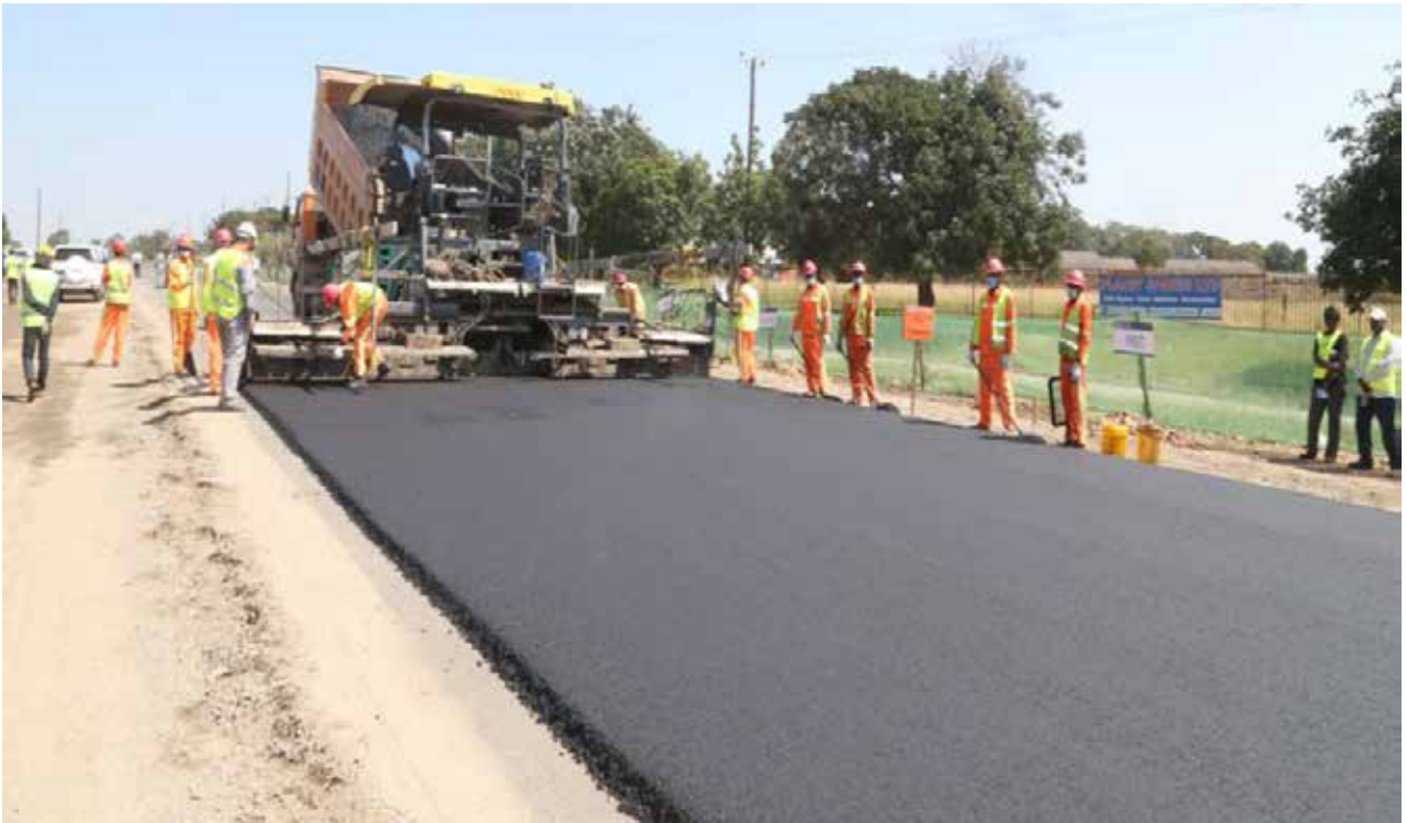
Figure 4: Rehabilitation works on the Kafue Mazabuka road Lot 1.
