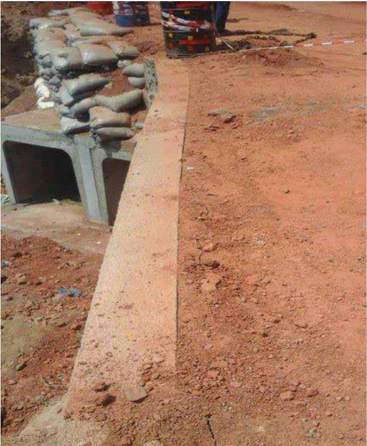
Figure 11: Final culverts at Ngozi
