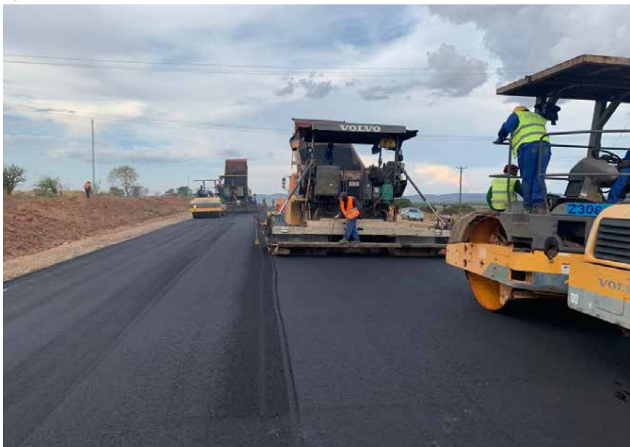
Figure 7: Rehabilitation of Turn Pike – Chikankata Turn off Road
