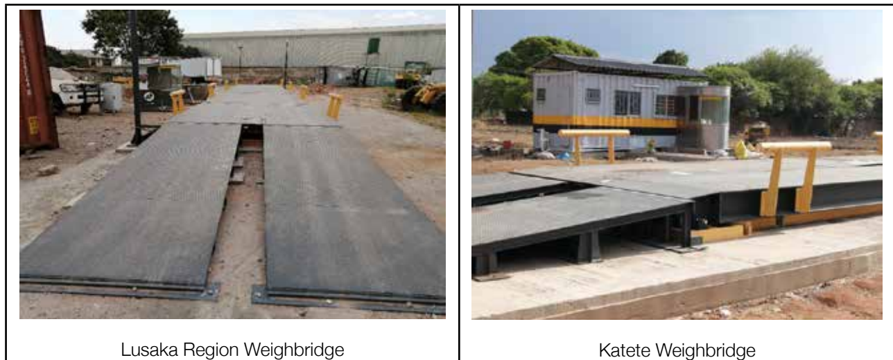
Figure 10: Weigh Bridges at two Locations
