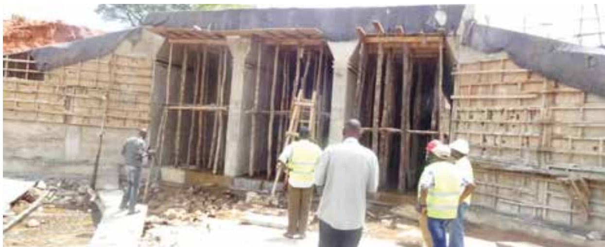
Figure 8: Lufune Box culvert under construction
