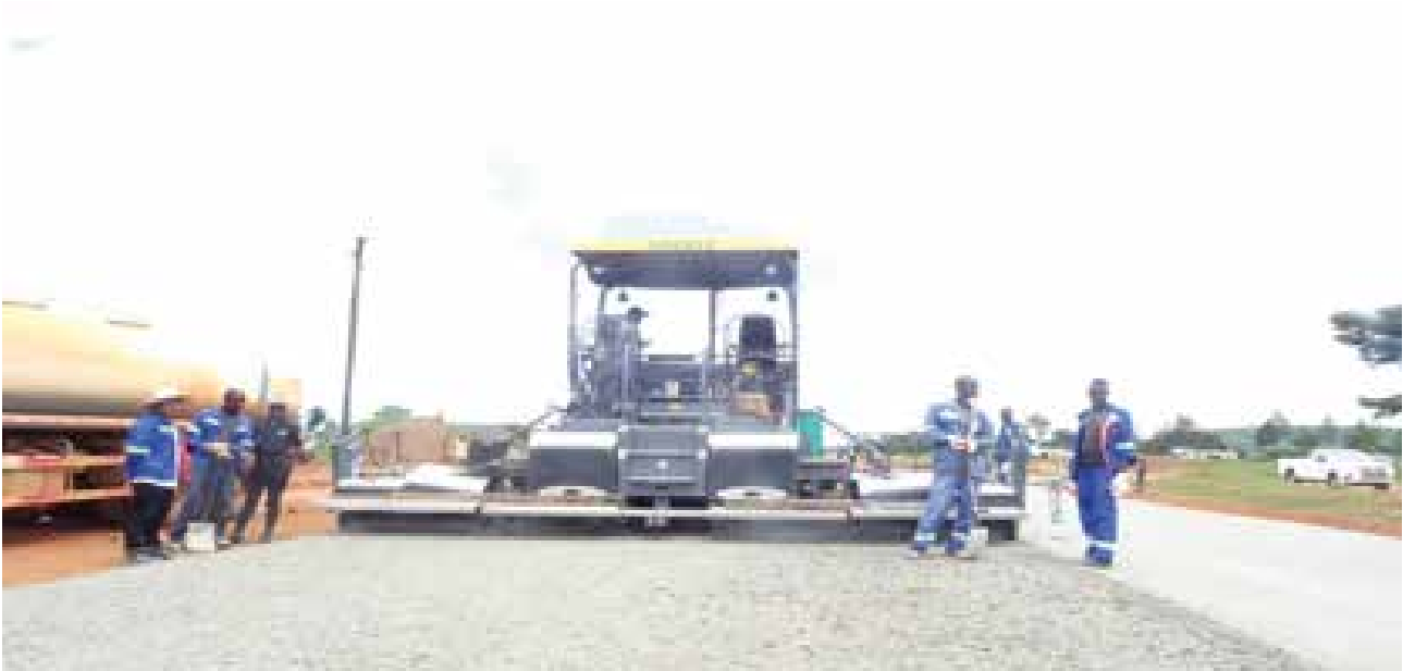
Figure 6: Rehabilitation works on the Chinsali-Nakonde road
