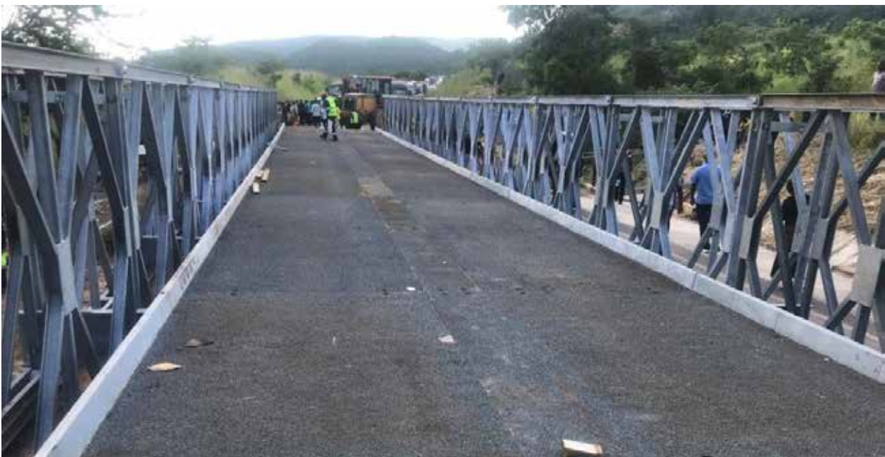
Figure 10: The Acrow Bridge which was mounted as a temporary measure at Ngozi Culvert
