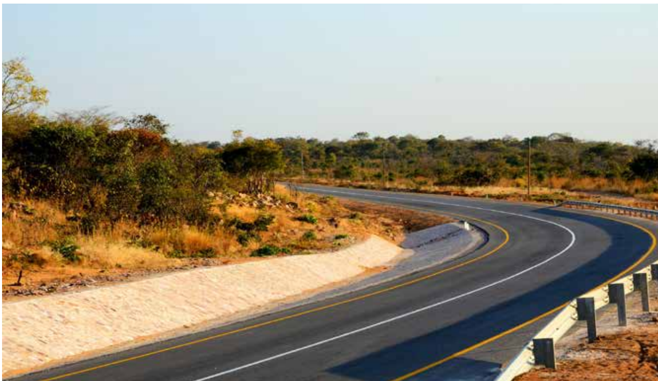
Figure 16: Rehabilitated Mansa-Luwingu road
