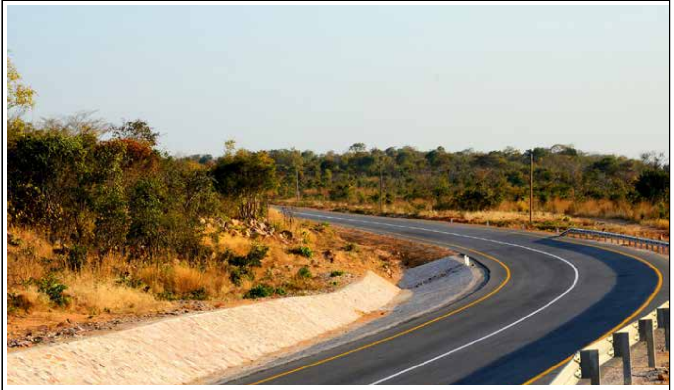
Figure 14: Rehabilitated Mansa-Luwingu road.
