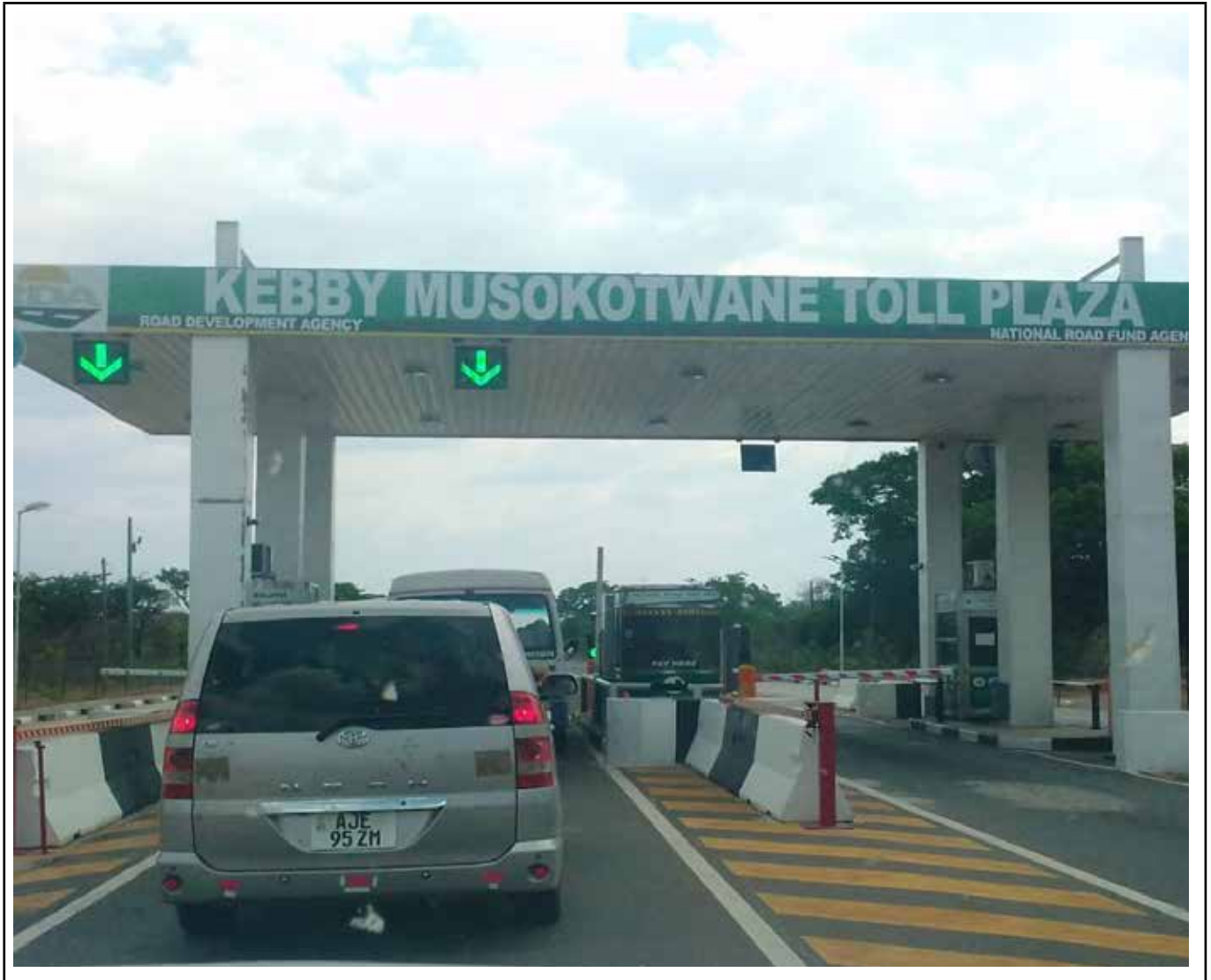
Figure 9: Kebby Musokotwane Toll Plaza on the Zimba-Livingstone Road.
