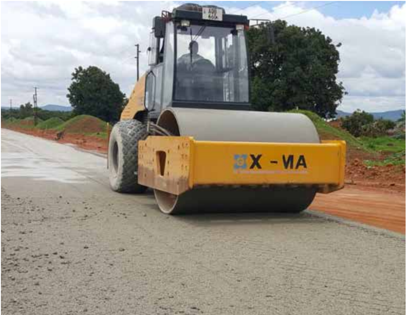
Figure 2: Rehabilitation works on the Chinsali-Nakonde Road.
