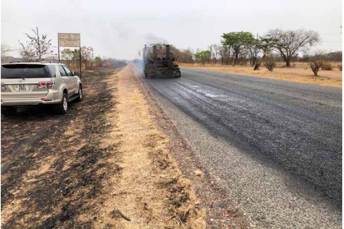
Figure 3: Armaseal trial on Mazabuka-Monze Road.
