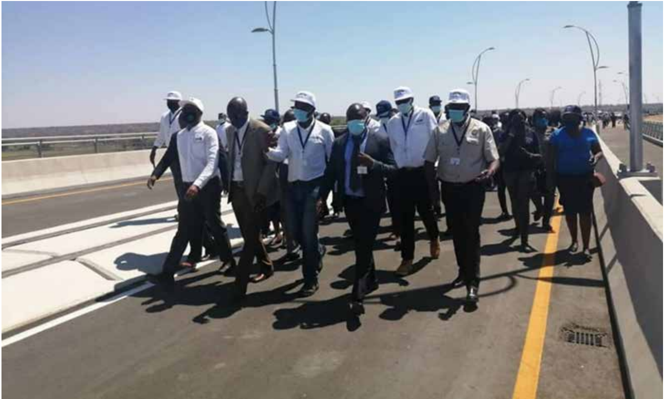
Figure 12: Final inspection of the Kazungula Bridge by Housing and Infrastructure Development Minister Hon. Vincent Mwale and his counterpart from Botswana Hon. Thulangano Segokgo on October 17, 2020.
