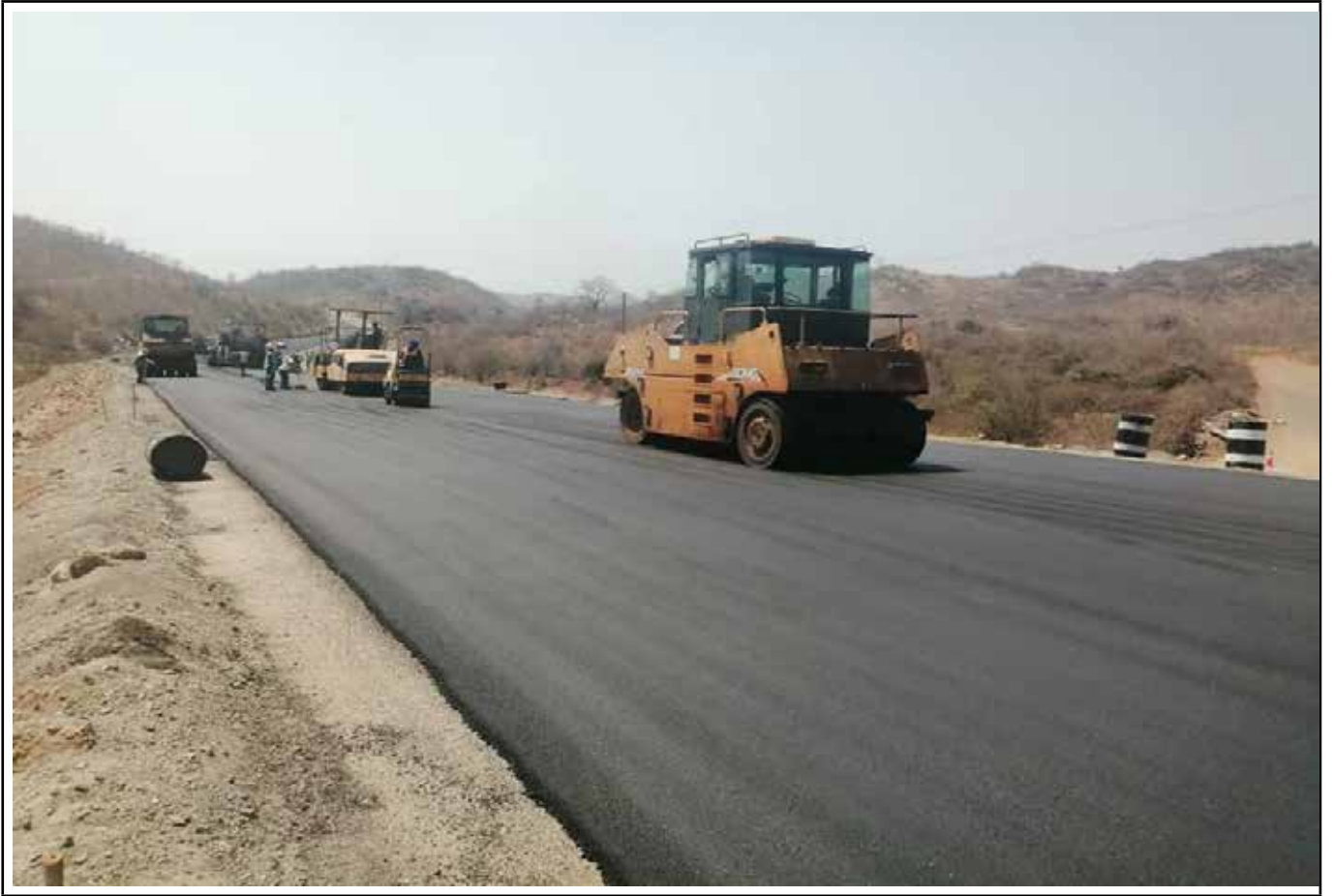
Figure 13: The rehabilitation works of the Turnpike-Mazabuka road.
