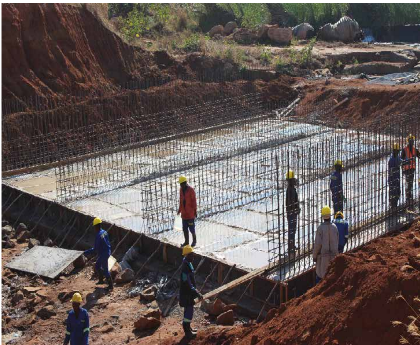
Figure 6: Msuzi bridge rehabilitation works
