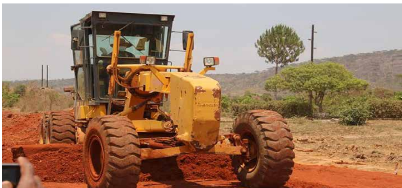
Figure 5: Feeder Road works
