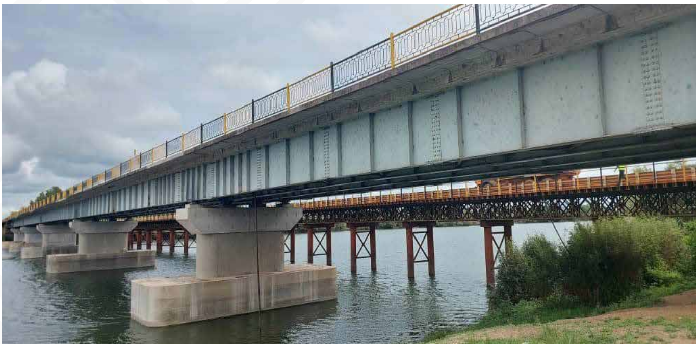
Figure 11: Rehabilitated Kafue Hook Bridge
