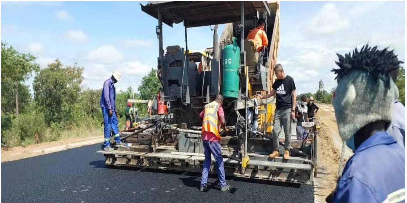
Figure 8: Mongu to Limulunga Road Works
