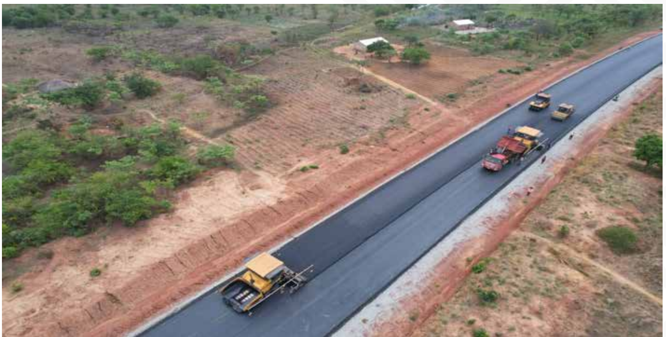
Figure 9: Chinsali to Nakonde Road Rehabilitation Works
