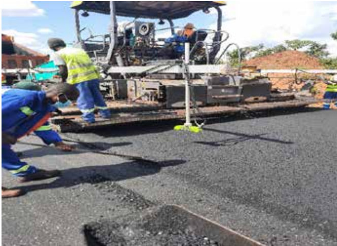
Figure 25: The RDA team checking whether the asphalt concrete surfacing on the Chinsali to Nakonde Road Lot 1 is of the right temperature as part of quality control and assurance during the vendor rating inspections
