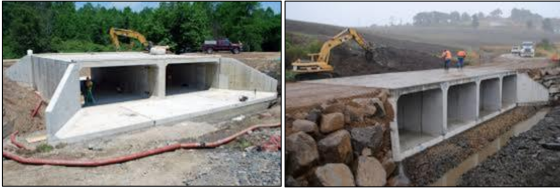
Figure 2-8: Monolithic structure – box culvert
