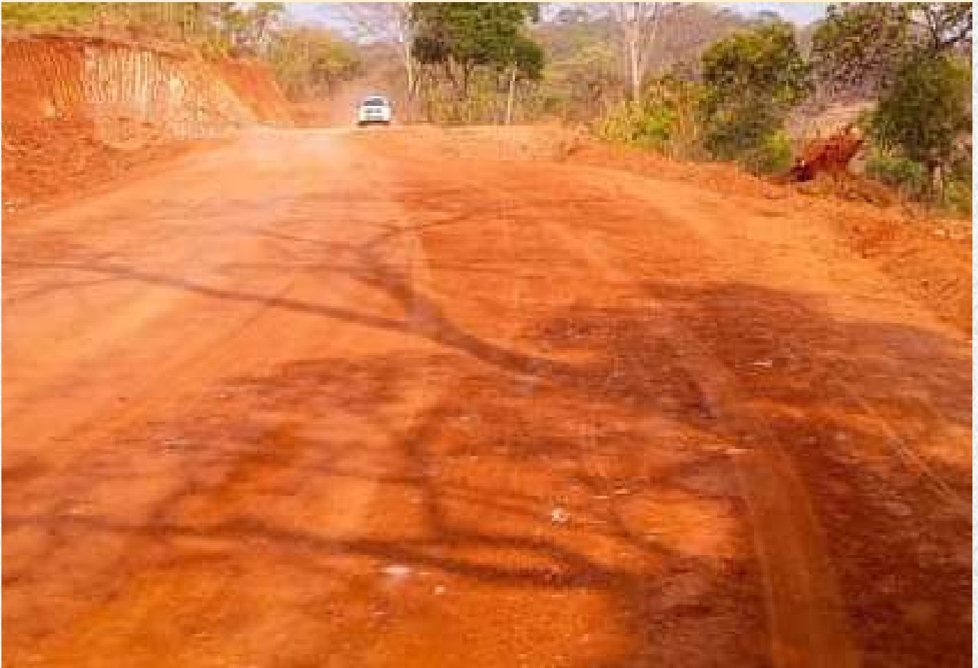
A section of the rehabilitated Chipata-Magwero Road in Eastern Province.
