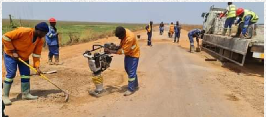
Pothole patching works on the Tuta Road.
