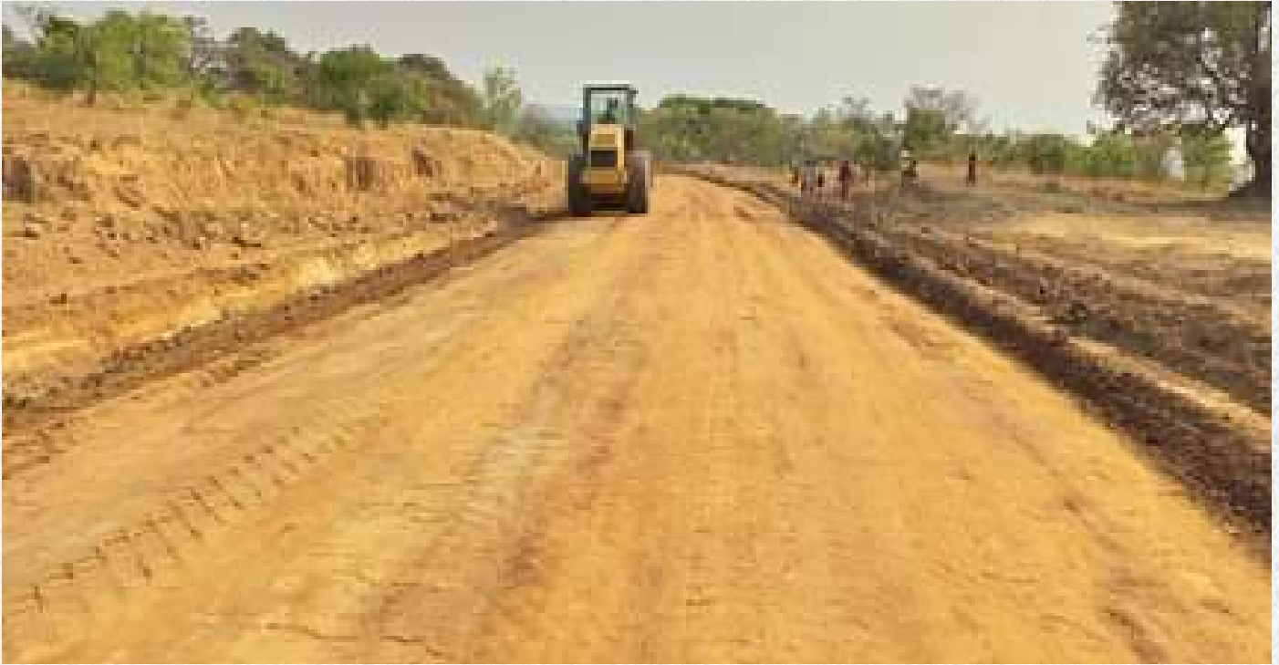
Re-graveling works on the Chipata-Vubwi Road.
