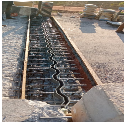
Preparation of Expansion Joint (Before)
