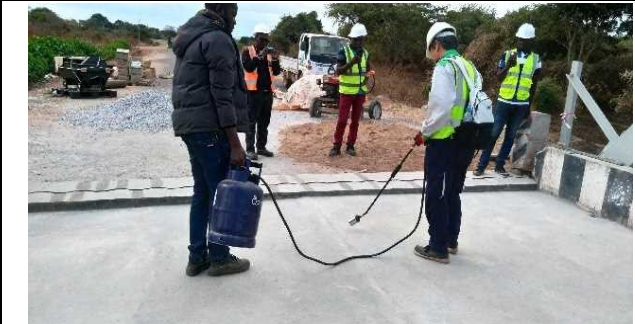
Fiber protrusion removal (using burner)
