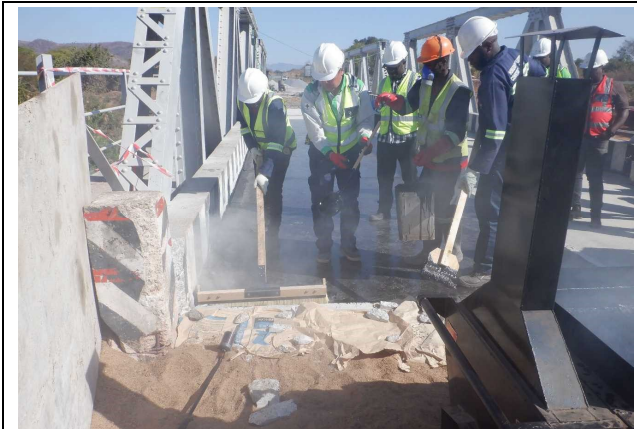
Waterproof layer application status
