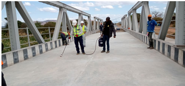
July 13: Technical Assistance: Torching of Protruding Fibers
