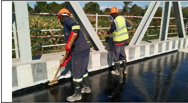
Waterproof layer application/work situation
