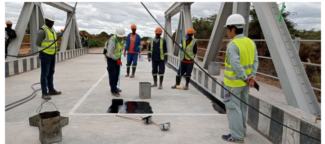
July 14: Technical Assistance: Application of Caticcoat Resin
