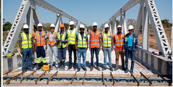
3 rd OJT on Bridge Repair @ Rufunsa Bridge
