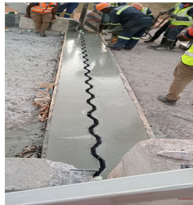
Photo of Expansion Joint (After)
