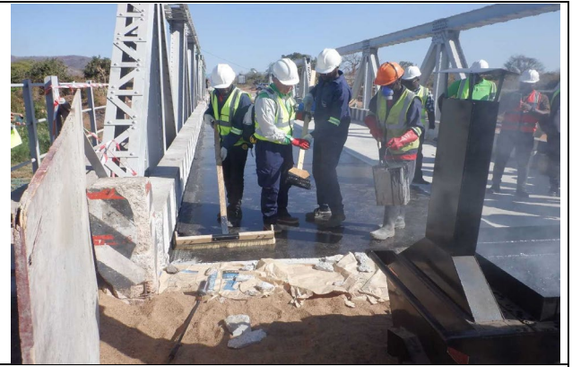
Waterproof layer application status
