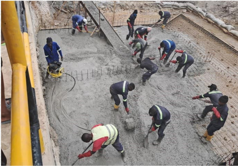
Construction works at the Gibson Chimfwembe and Lulamba box culverts in Chingola District.
