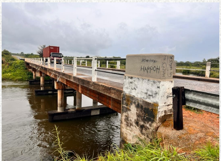
Lukulu Bridge along the Kasama-Luwingu Road.
