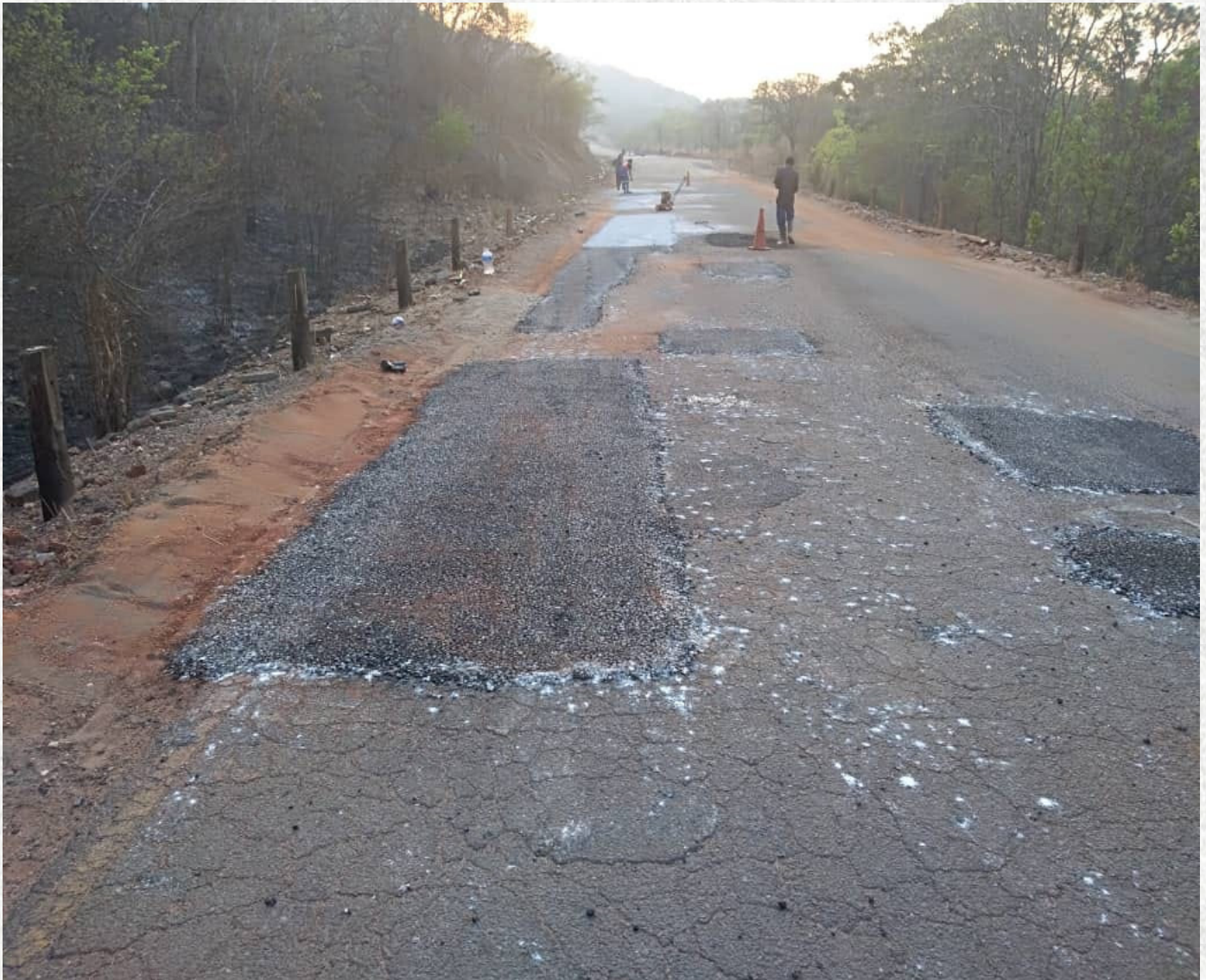
Pothole patching along the Great East Road (Lusaka -Luangwa Road section).
