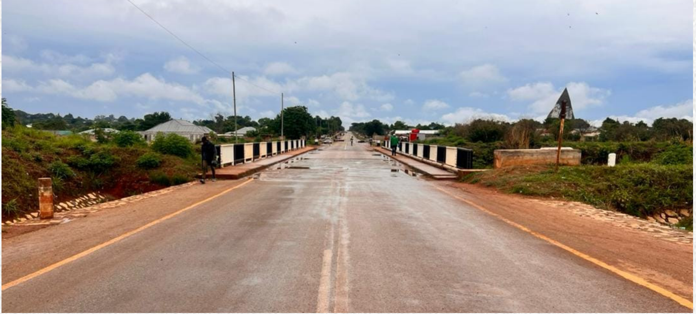
Lukashya Bridge in Kasama District.
