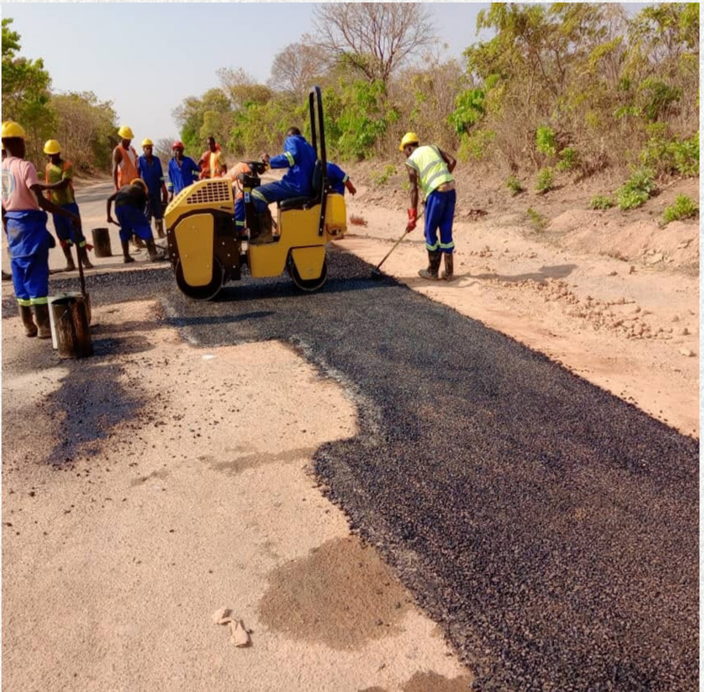
Lundazi-Chasefu Road in Eastern Province.
