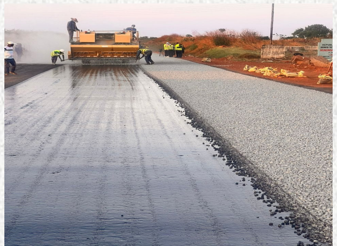
Reconstruction works on some sections of the Great North Road.
