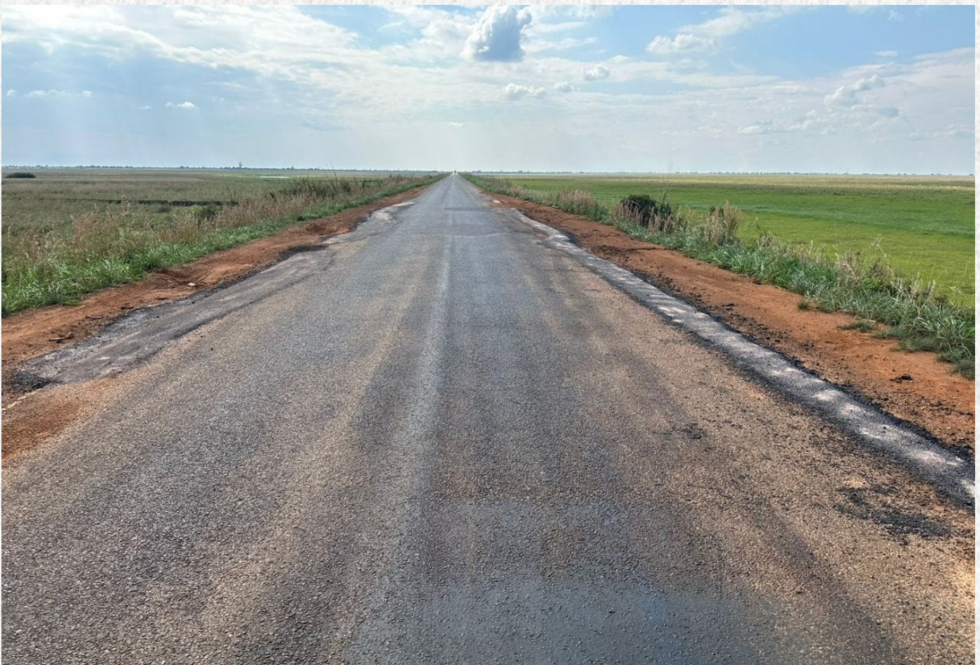
Edge repair works on the Tuta Road.
