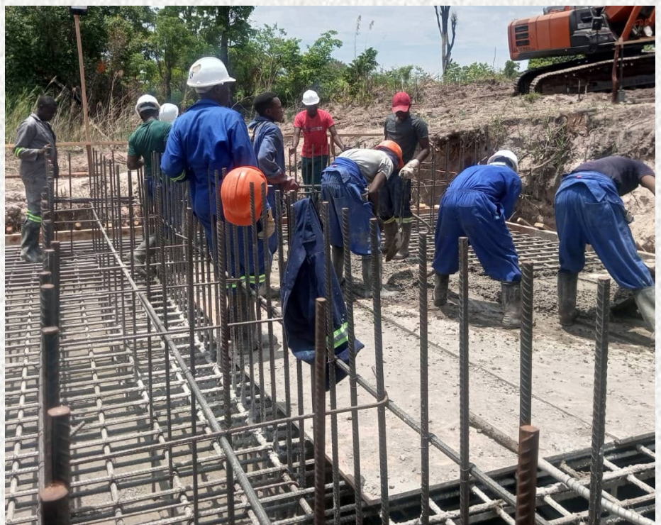
Ongoing construction works of the Aluni Mulonga ACROW Bridge.
