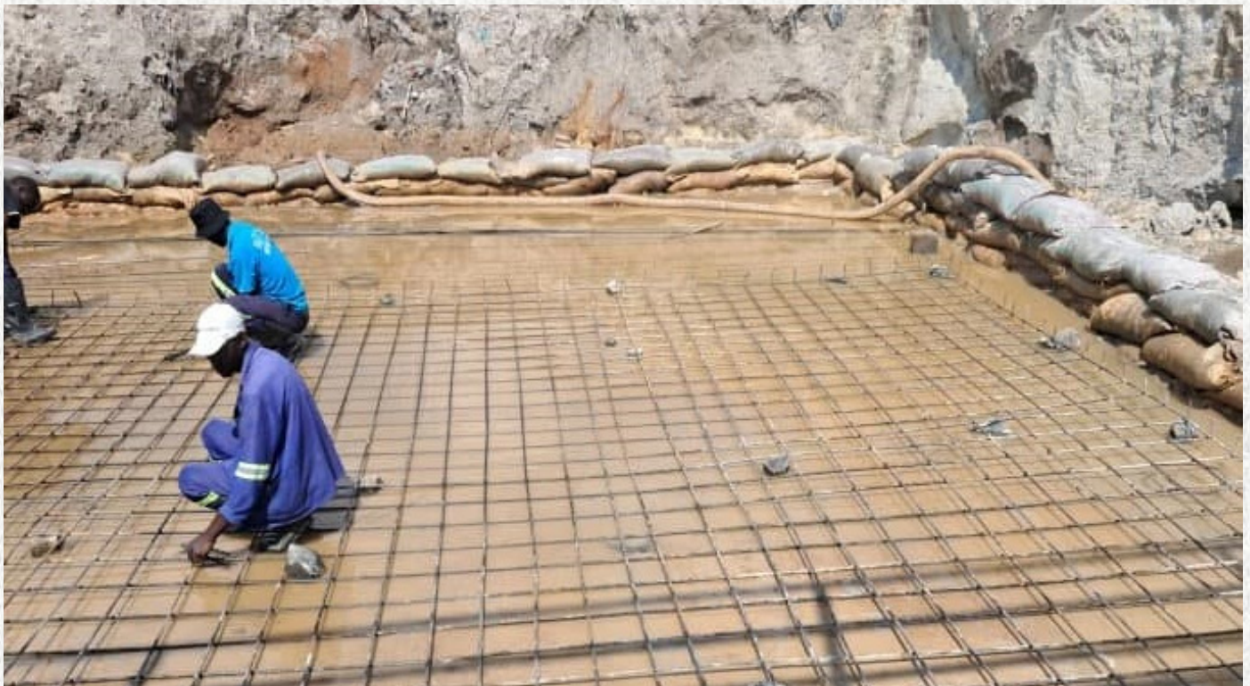
Steel enforcement on Gibson Chimfwembe and Lulamba box culverts.
