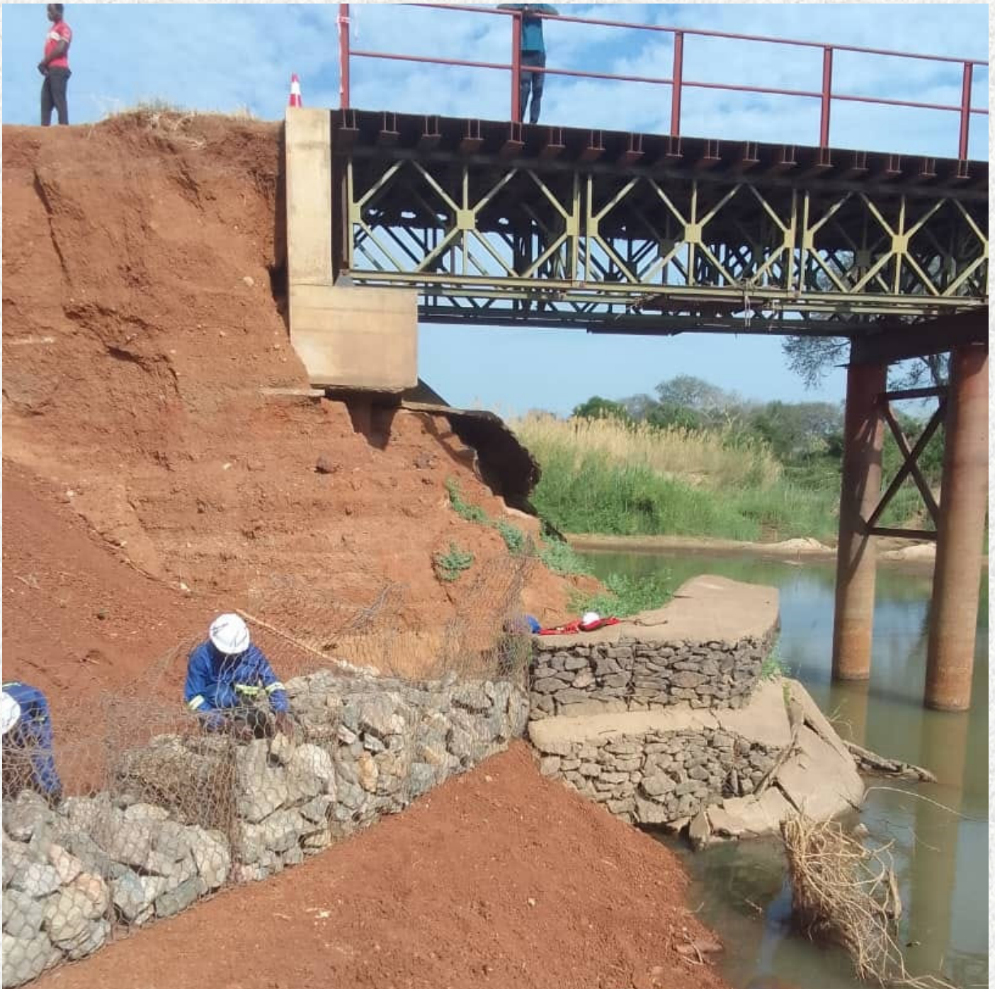
Emergency maintenance works on Luangwa Bridge along the Chama-Matumbo Road.
