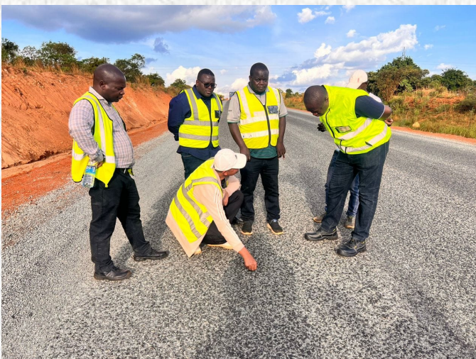
Checking on the pavement structure.
