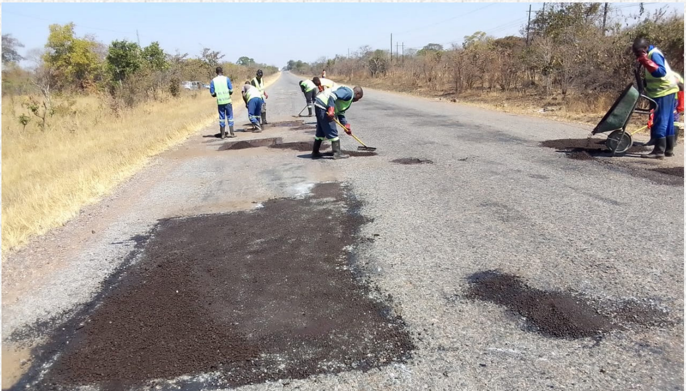
Pothole patching works on the Monze-Mazabuka Road.
