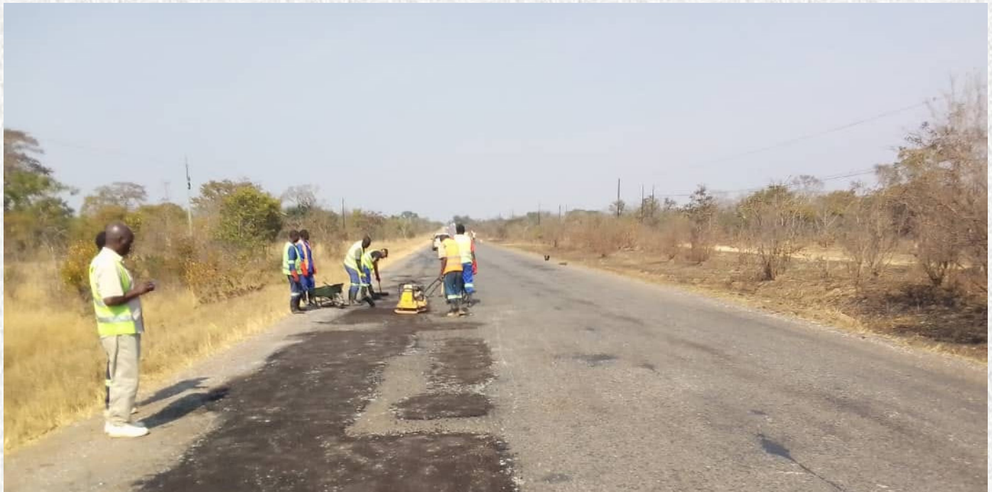
Pothole patching works on the Monze-Mazabuka Road.
