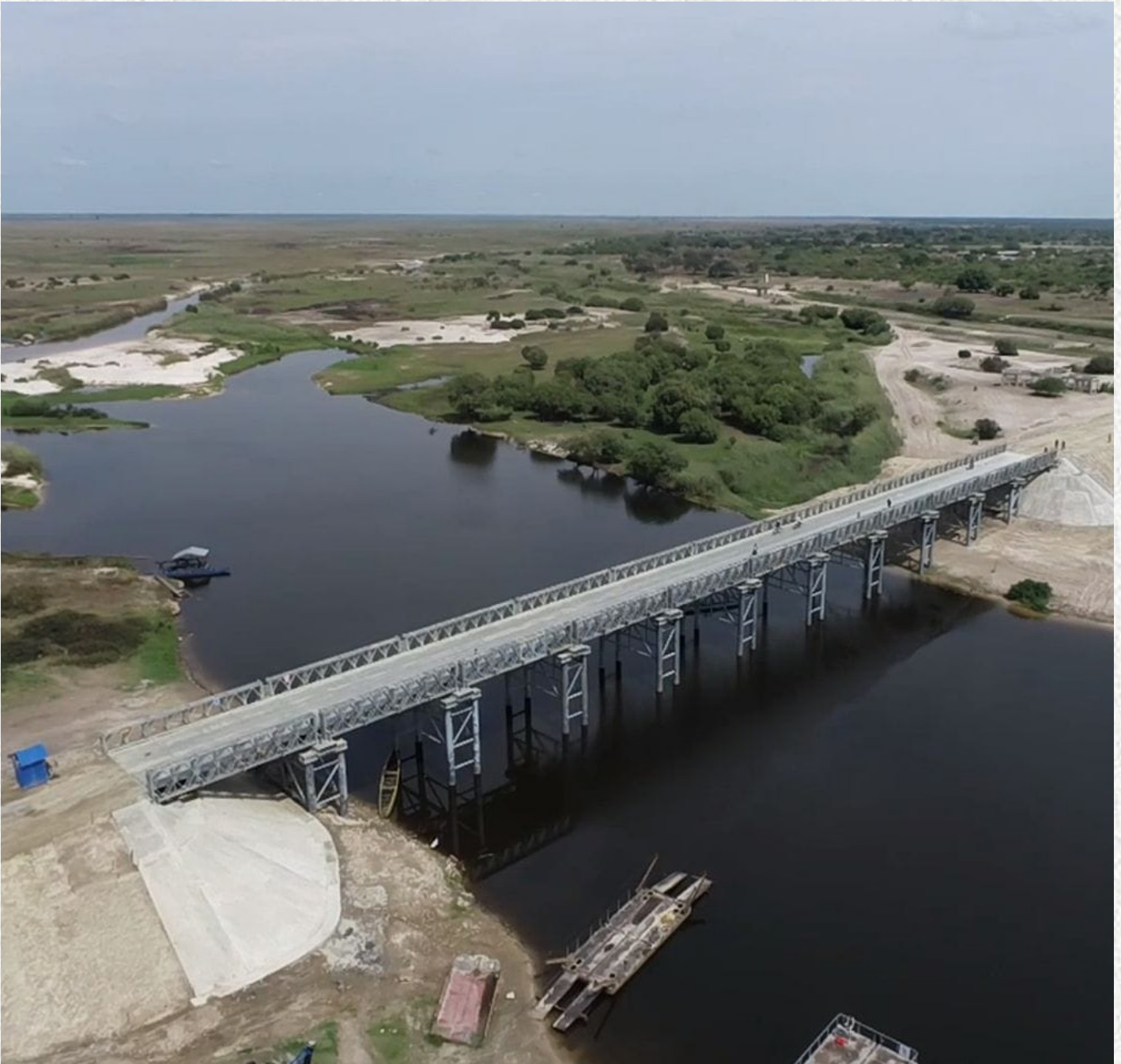
Newly constructed Luanginga Bridge in Kalabo District in Western Province.
