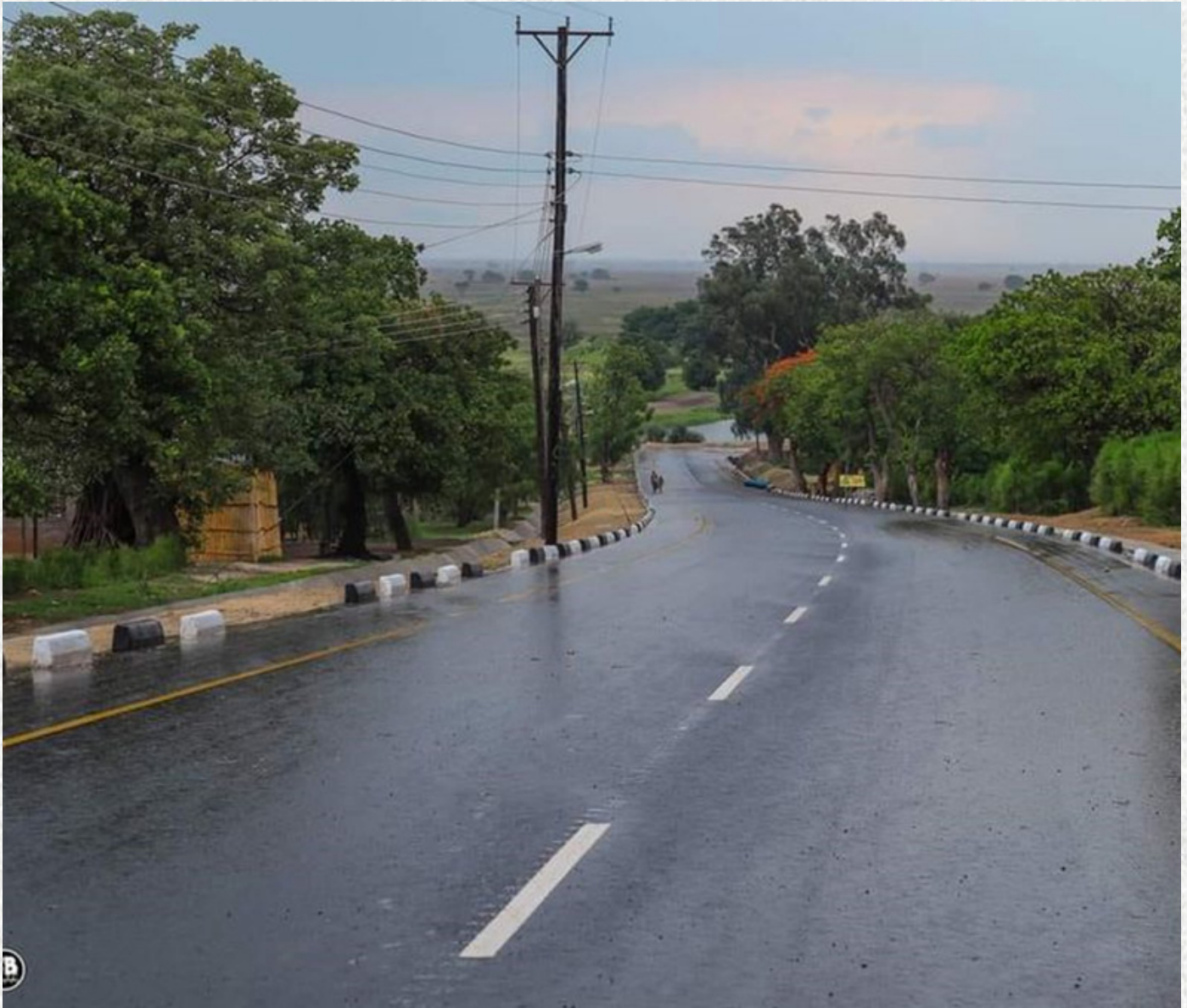
Newly rehabilitated Mongu-Limulunga Road.
