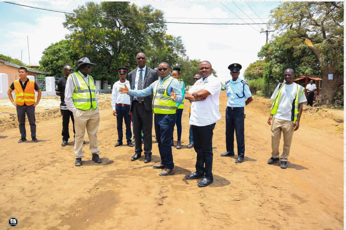
RDA Western Regional Manager, Eng. Paul Habasimbi (gesturing) updating Infrastructure, Housing and Urban Development Minister, Hon. Eng. Charles L. Milupi (far left) on the road works being undertaken in Mongu District.
