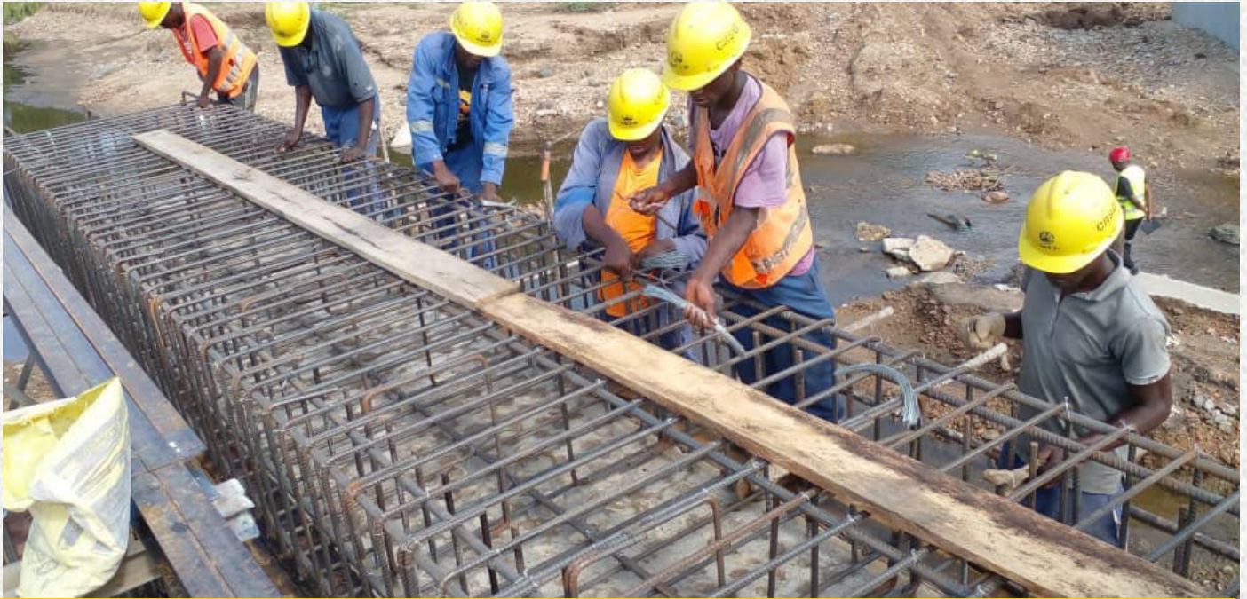
Steel works underway at Kampemba Bridge.
