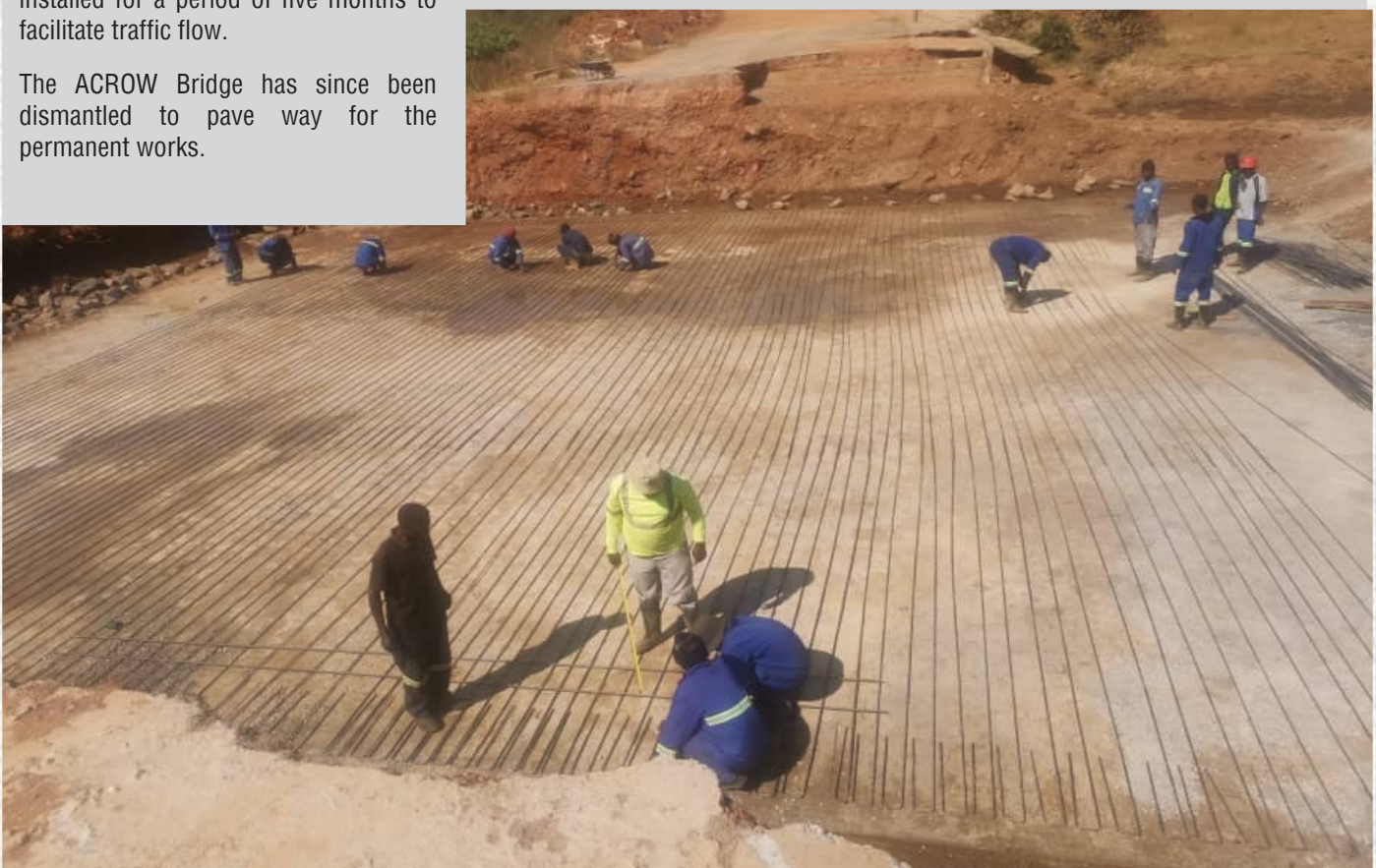
Blinding concrete works.
