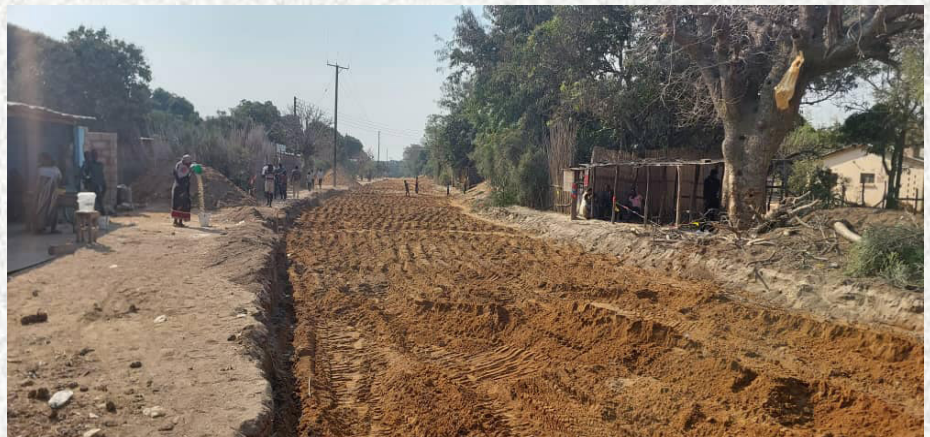
Extension works of the Mongu-Limulunga Road.
