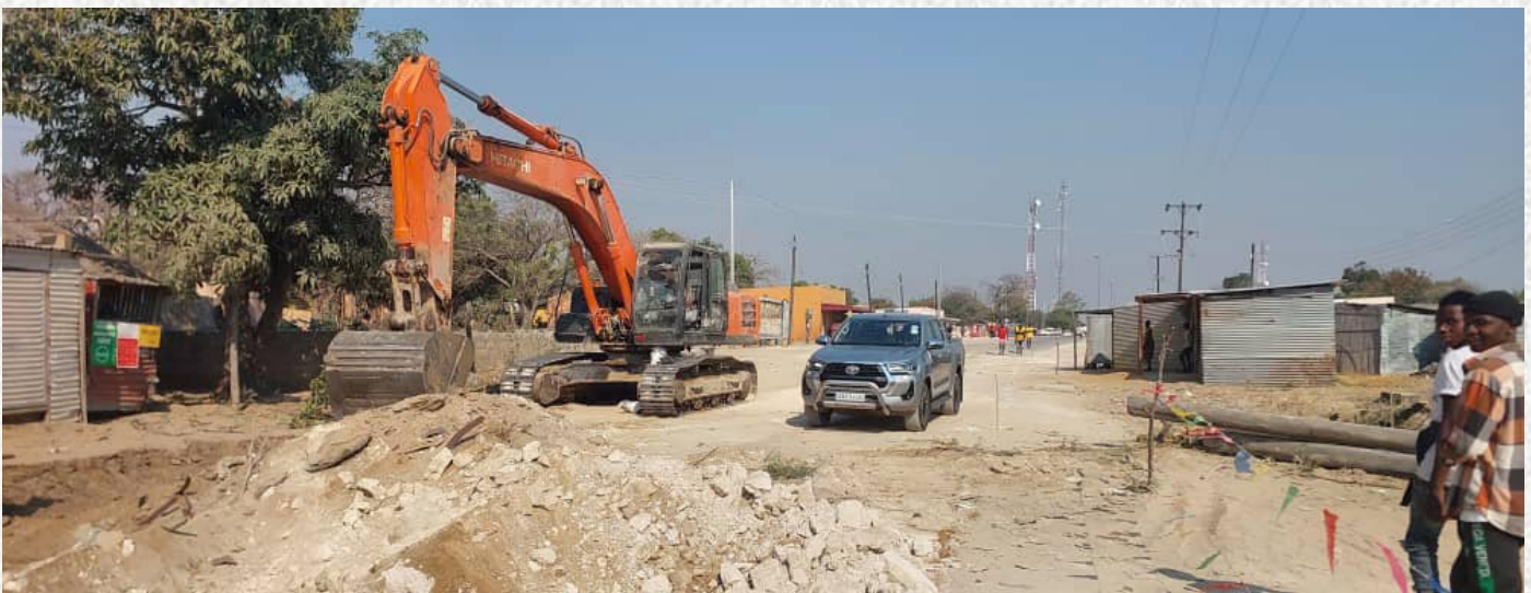
Excavation works in progress.
