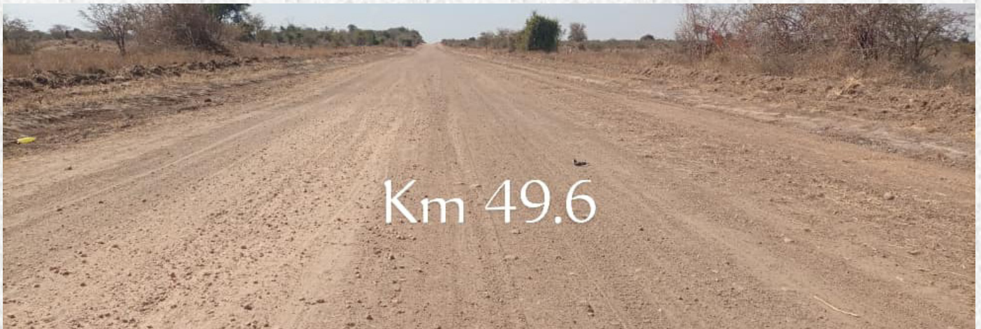
Re-gravelled section.
