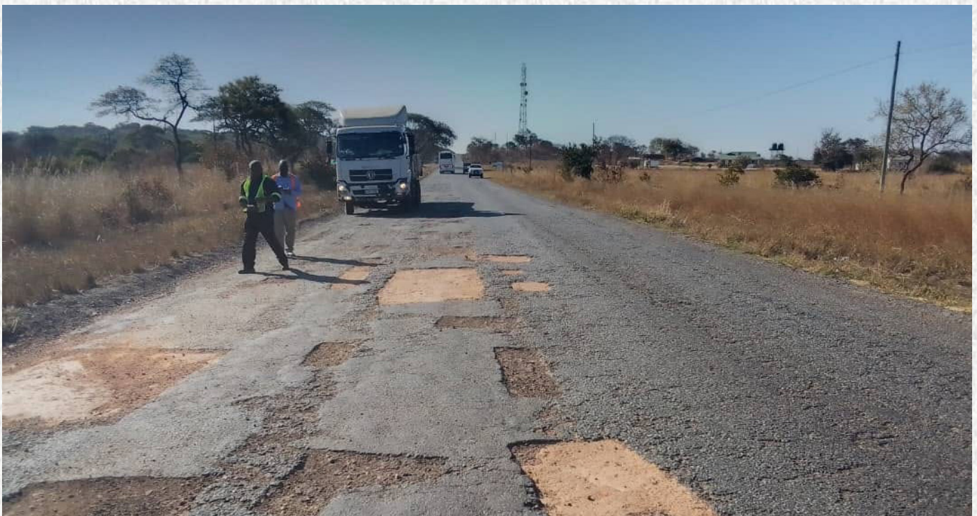
Pothole shaping works.
