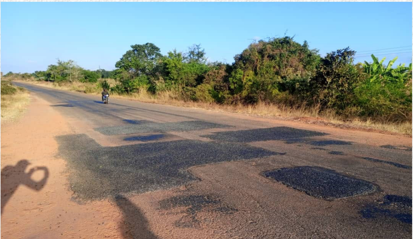
Patched section of the Chiptata-Mfuwe Road.
