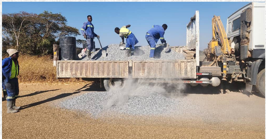
The truck offloading road aggregates.
