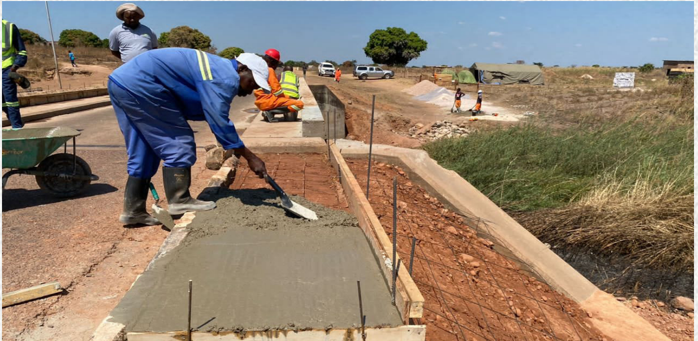
Kazembe Twin Bridges maintenance works on.
