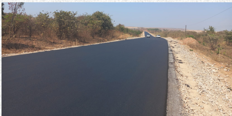
A completed section of the Chingola-Kasumbalesa Road.
