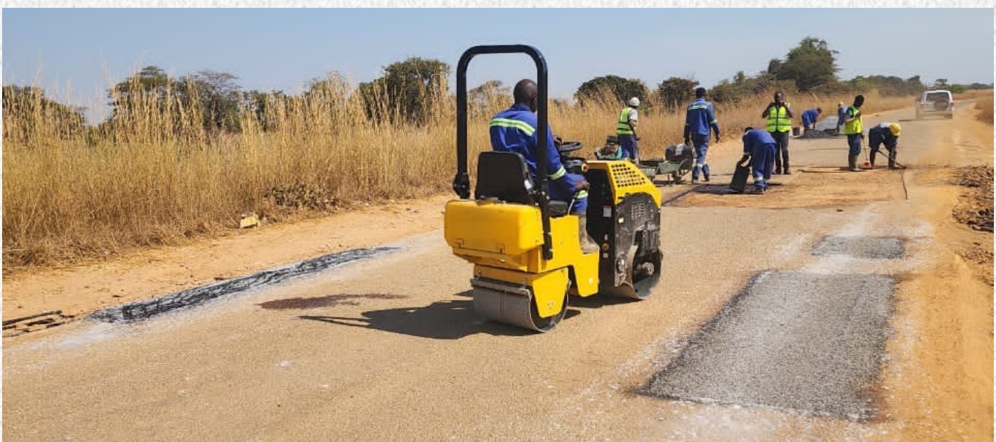
Pothole patching works in progress.
