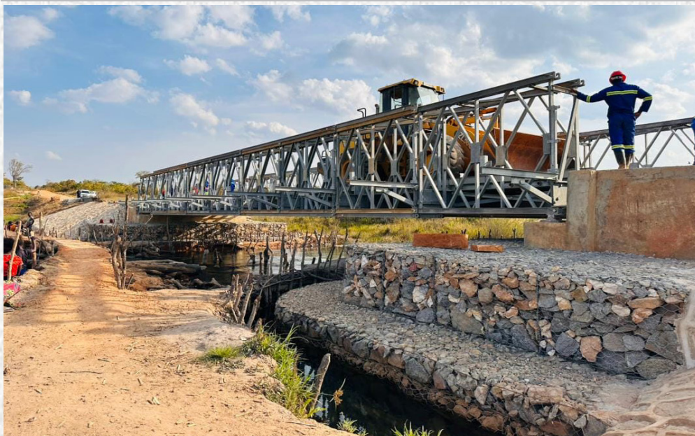
Completed Lukulu ACROW Bridge.
