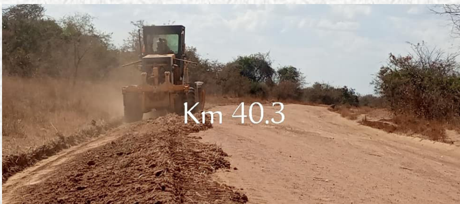
Road formation works in progress.
