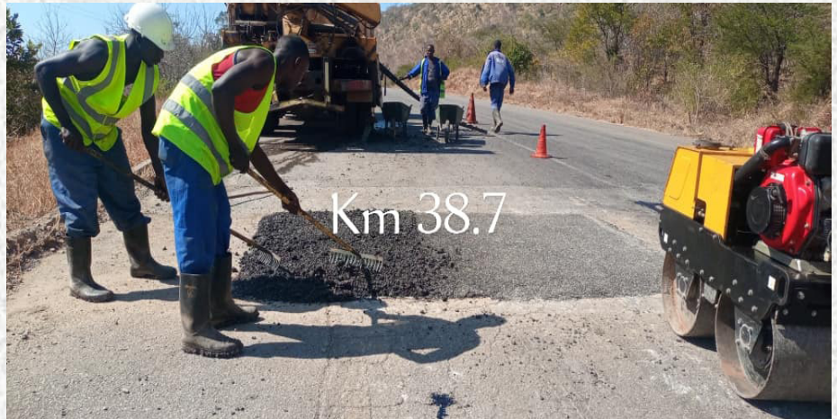
Pothole patching in progress.
