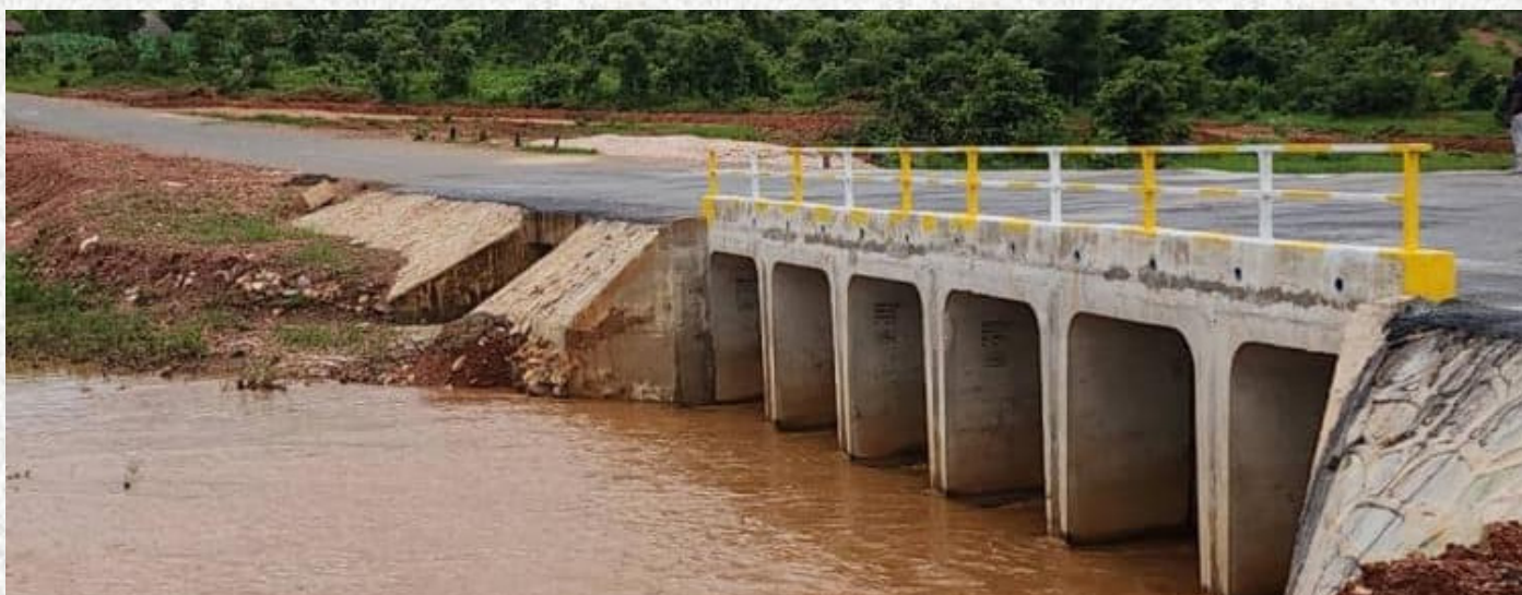
Newly constructed six lines of 2400 x 2400 millimeters portal culvert at Chiwena along the Mumbwa to Landless Corner Road in Central Province.
