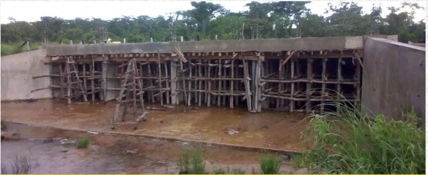
Construction works on the 3 X 2 metres insitu concrete box culvert along the Mporokoso-Mununga Road.
