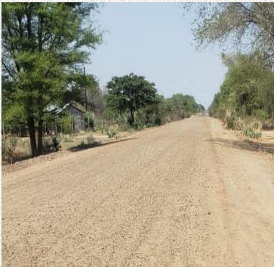
The section of the Kazungula-Sesheke Road reconstructed to cement stabilized base.
