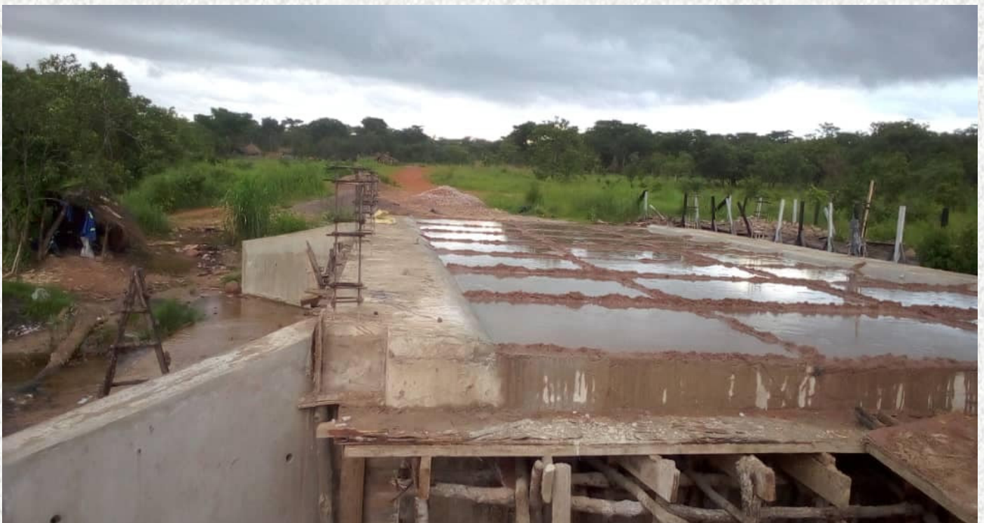
Works on the 3 X 2 metres insitu concrete box culvert along the Mporokoso-Mununga Road.
