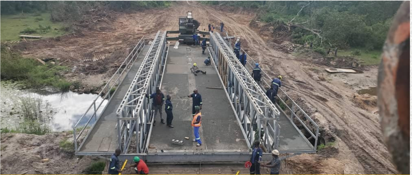
Malolwa ACROW Bridge under construction in Kabompo District in North-Western Province.
