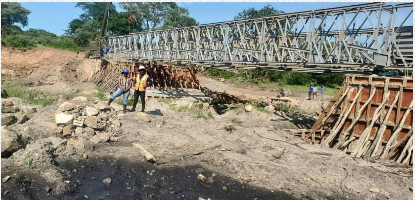
Malolwa ACROW Bridge under construction.
