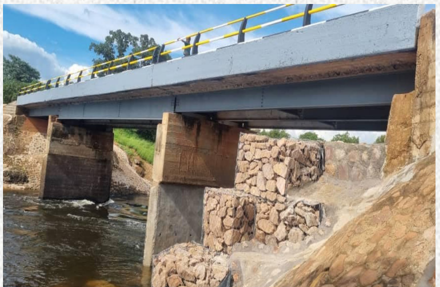
Gabion baskets fitted at Mukonshi Bridge in Chipili District.
