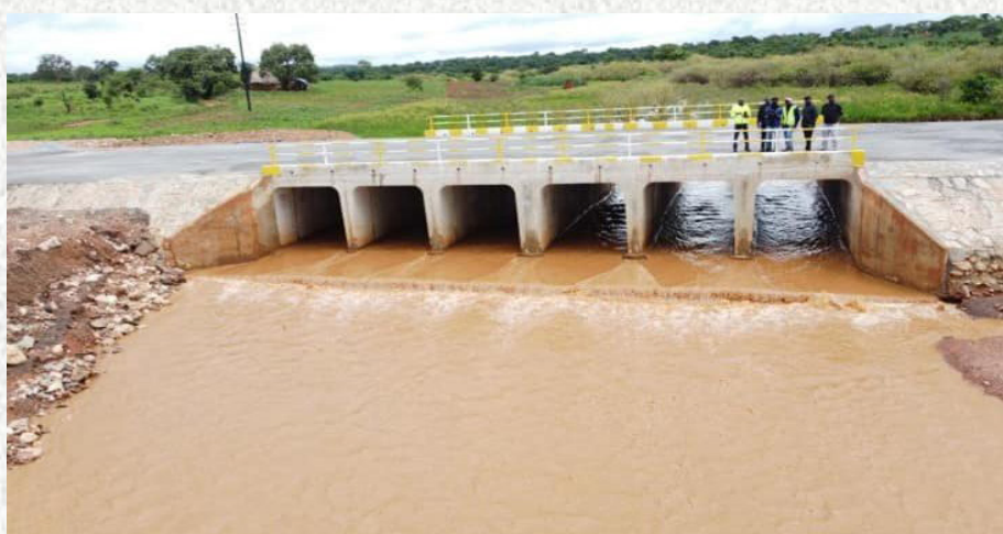
Six lines of 2400 x 2400 millimeters portal culvert at Chiwena along the Mumbwa to Landless Corner Road.
