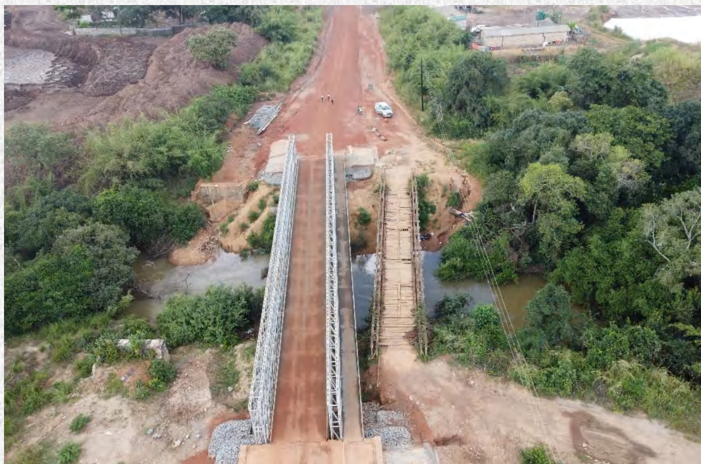
Newly installed Luombwa ACROW Bridge across the Luombwa River in the Nasanga Farm Block of Serenje District.
