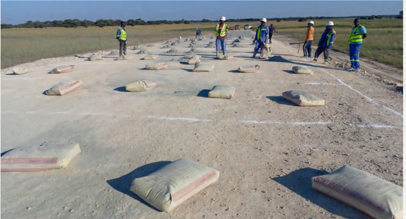
Preparations to commence cement stabilization .
