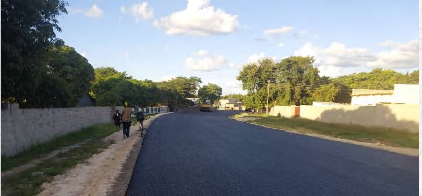
Asphalt concrete surfacing works on the Lyambai Road in Mongu District.
