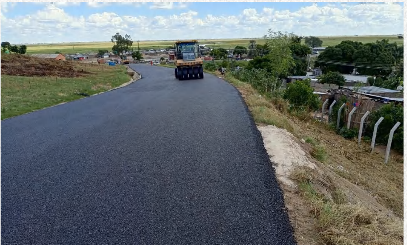
Asphalt concrete surfacing works on the Lyambai Road.
