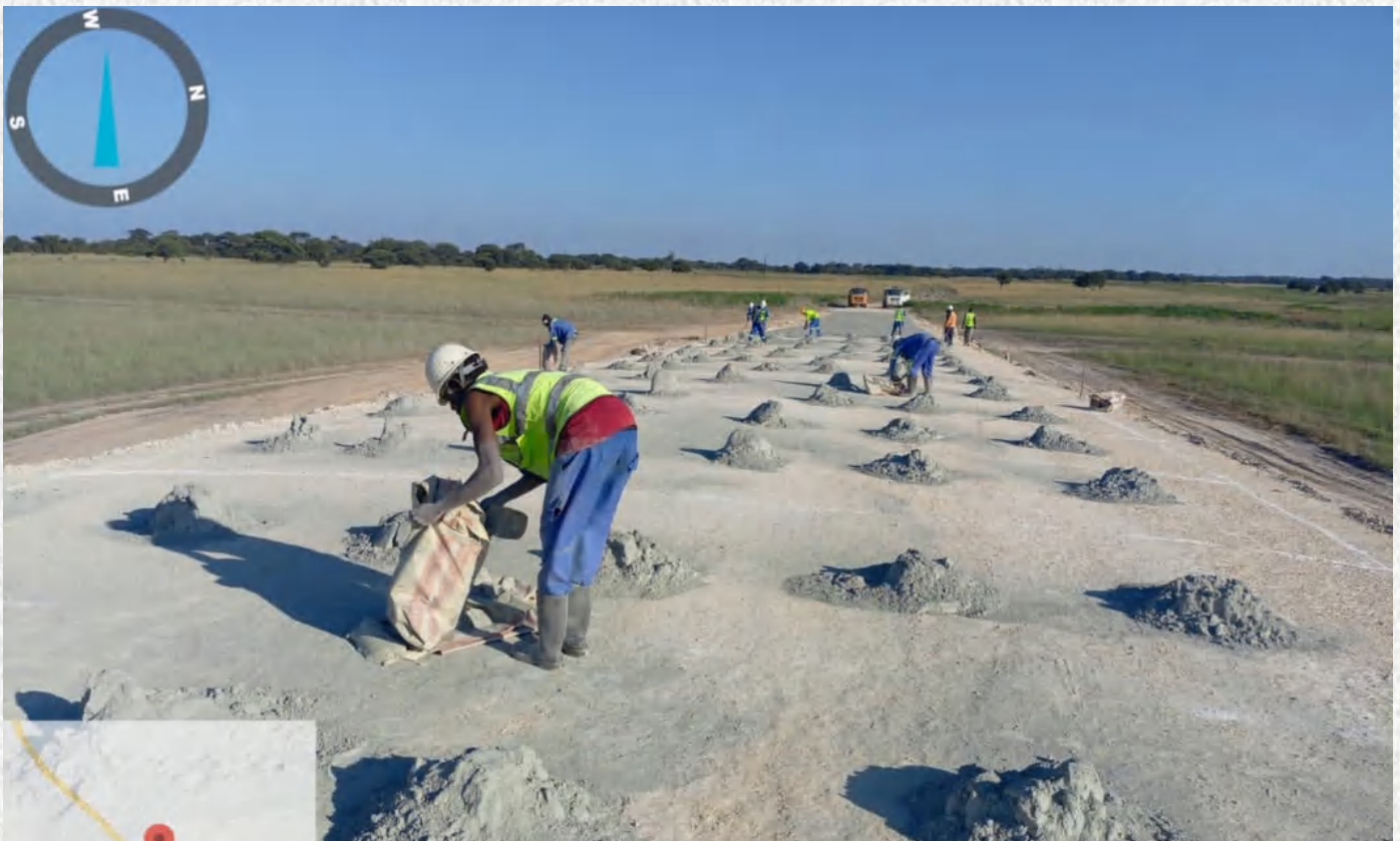
Preparations to commence cement stabilization.
