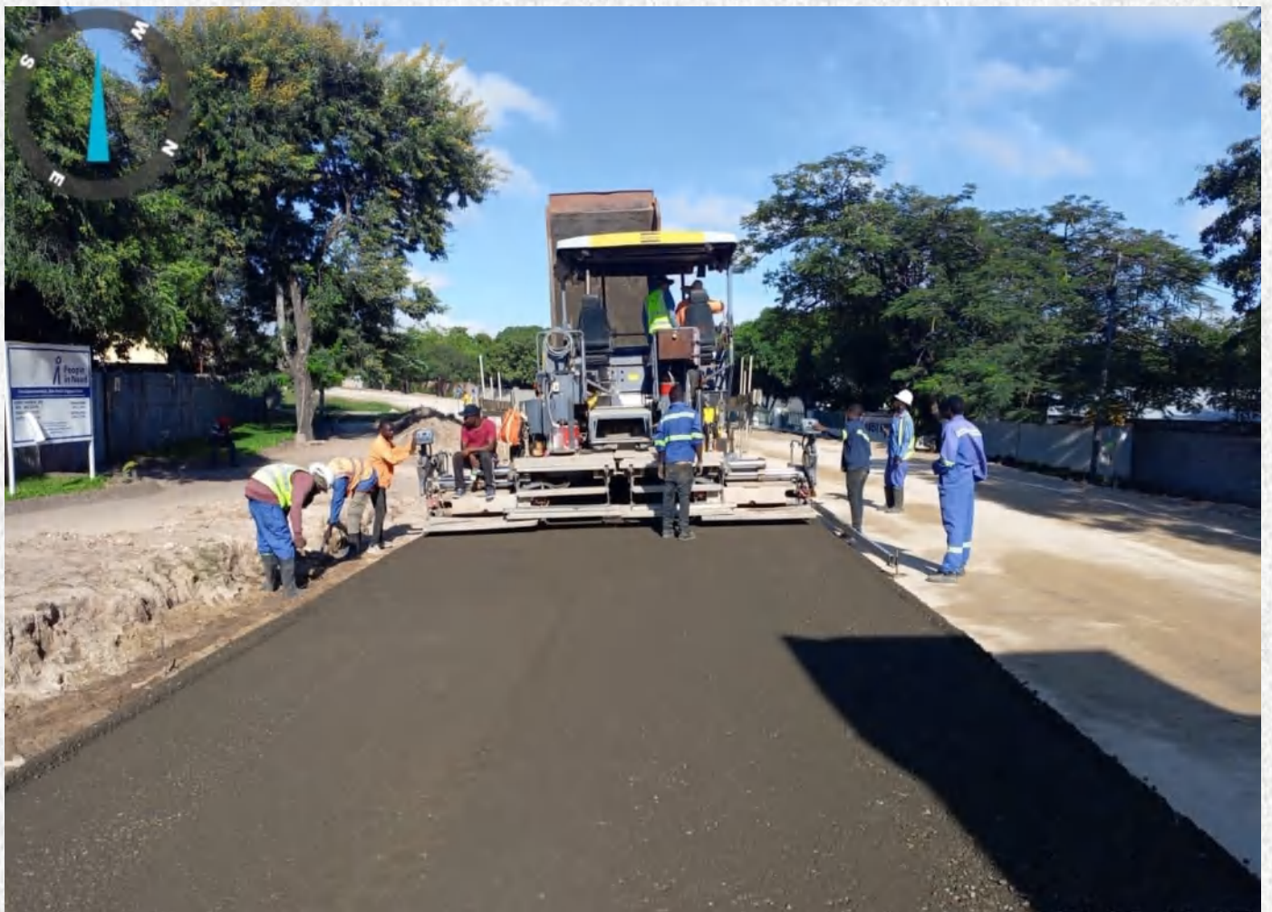
Laying of 175 millimetres crushed stone base on Lyambai road in Mongu.
