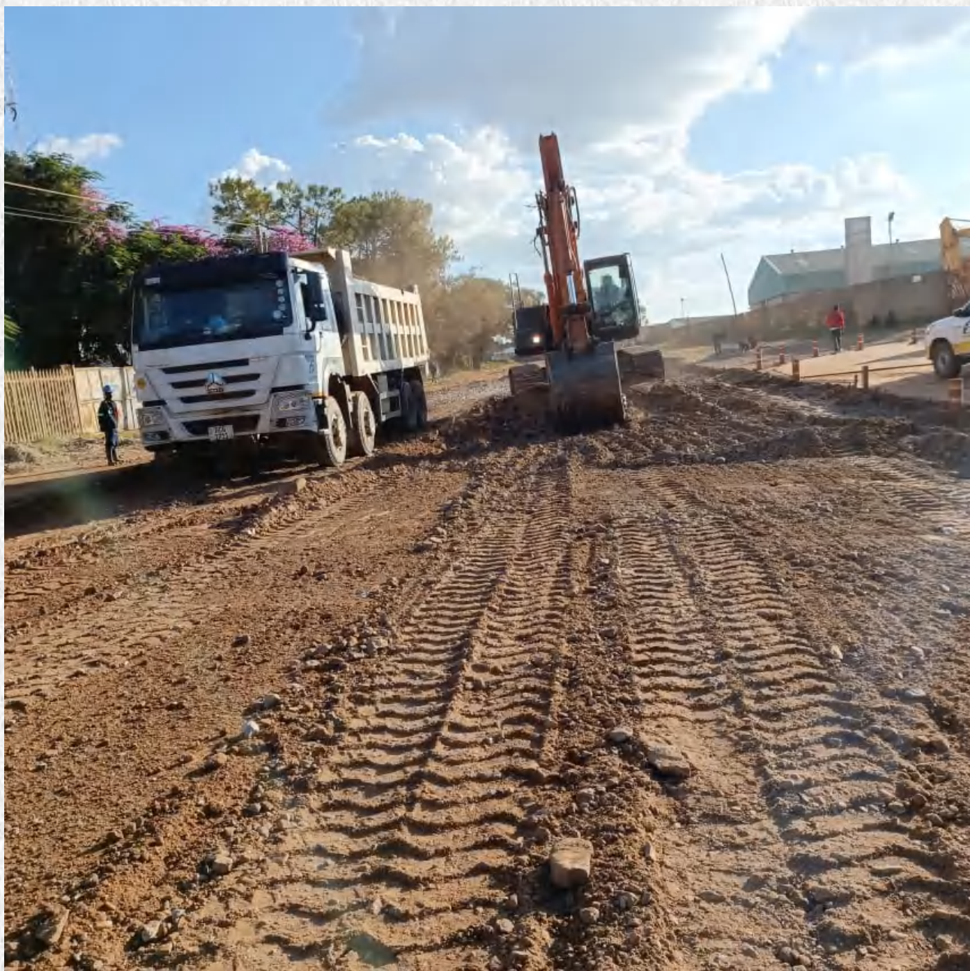
Clearing and grubbing works underway.
