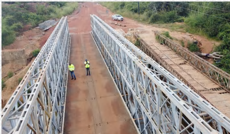
Newly installed Luombwa ACROW Bridge across the Luombwa River in the Nasanga Farm Block of Serenje District in Central Province.
