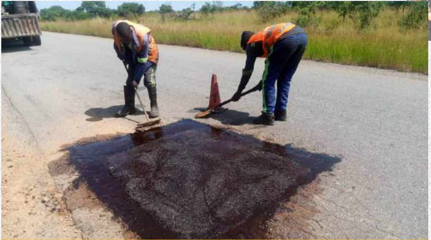
Pothole patching works in the Kafue National Park from the Nalusanga Gate to Tateyeyo Gate.
