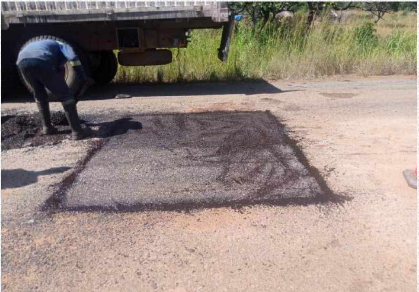
Pothole patching works in the Kafue National Park from the Nalusanga Gate to Tateyeyo Gate.
