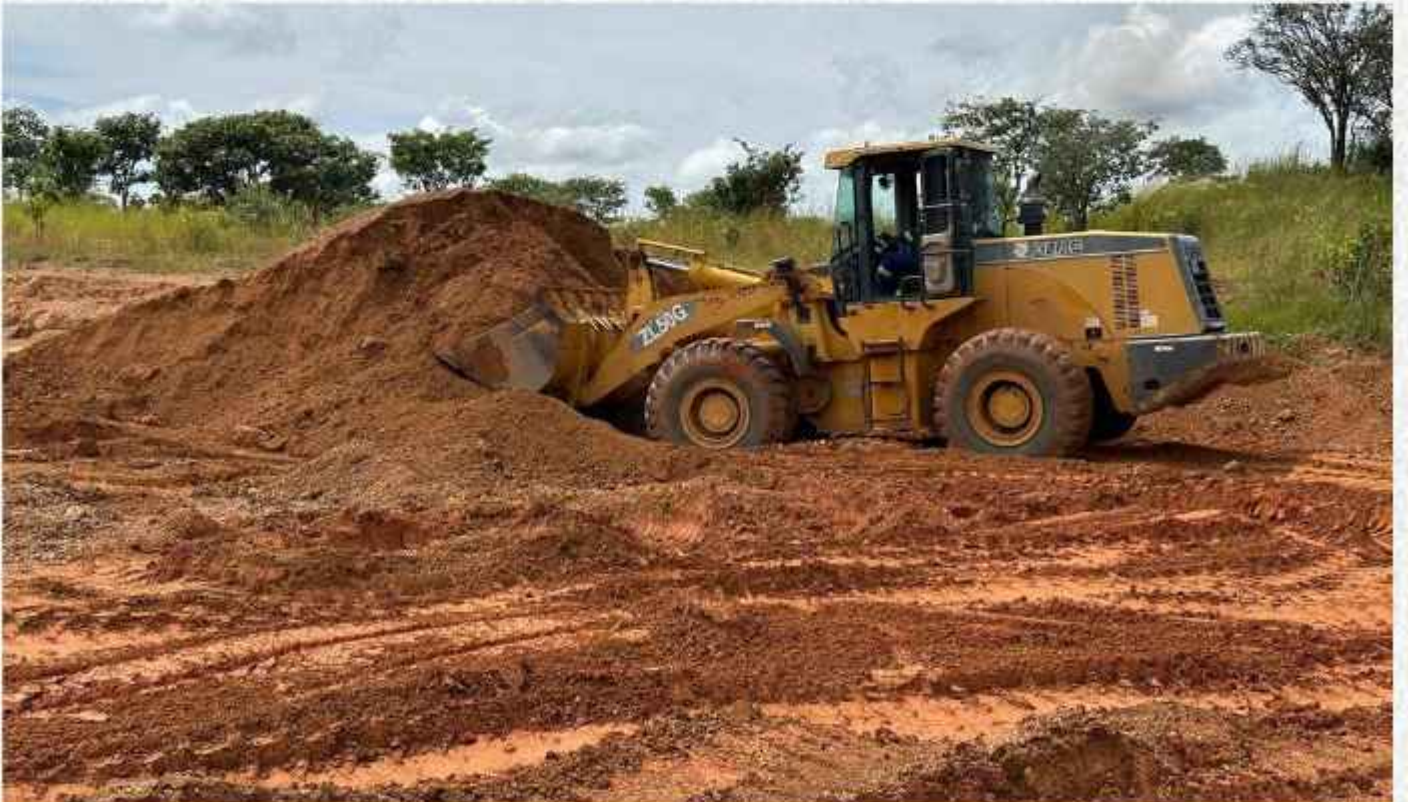
Holding maintenance works on the Musaila-Tuta Road.
