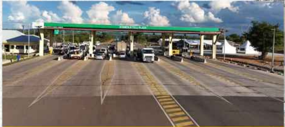
The newly constructed Konkola Toll Plaza along the Chingola-Kasumbalesa Road.
