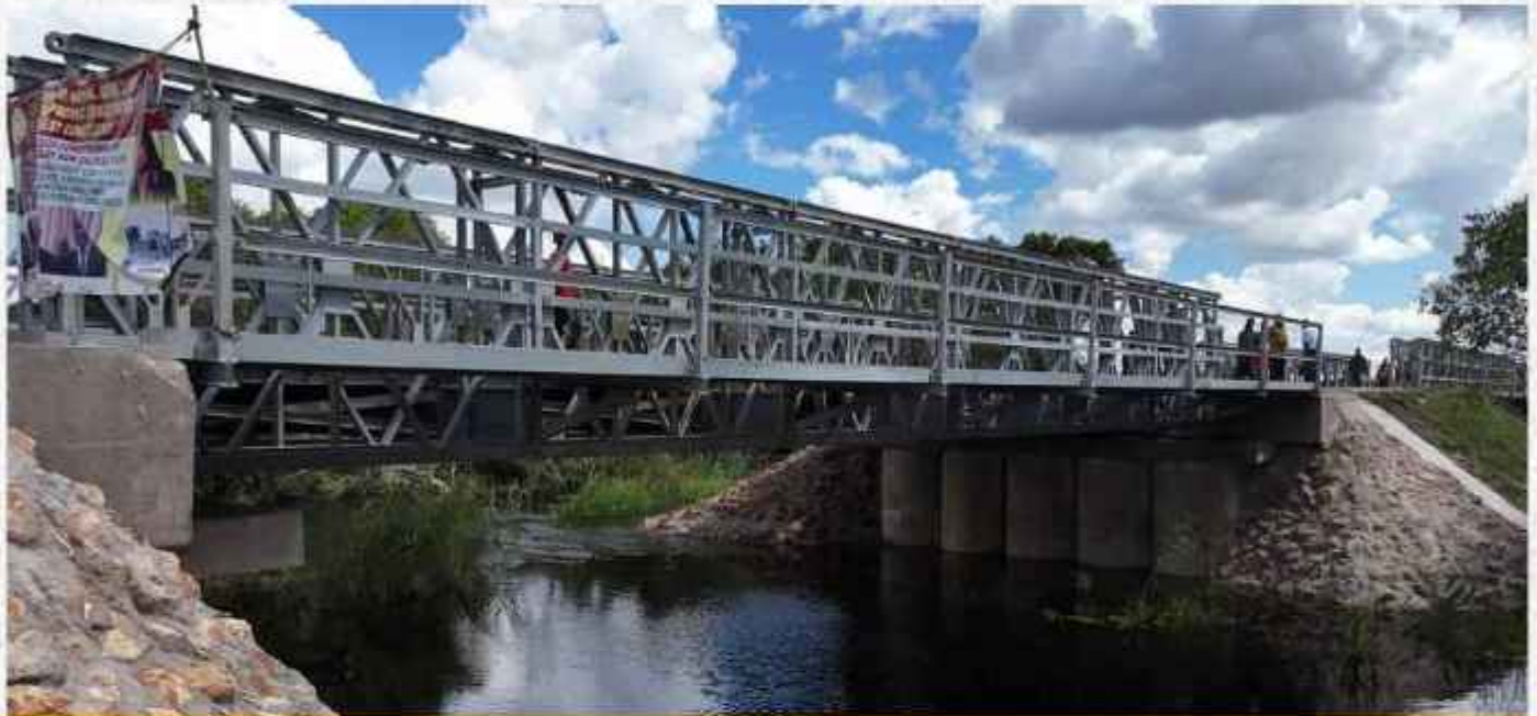
One of the commissioned ACROW Bridges across the Kashiji River along the Zambezi-Chinyama-Litapi Road in Zambezi District.
