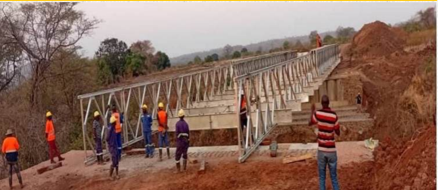
During the construction of the Lusangazi Bridge.
