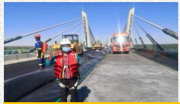
Eng. Kaulu supervising paving of the Kazungula bridge surface in 2020.
